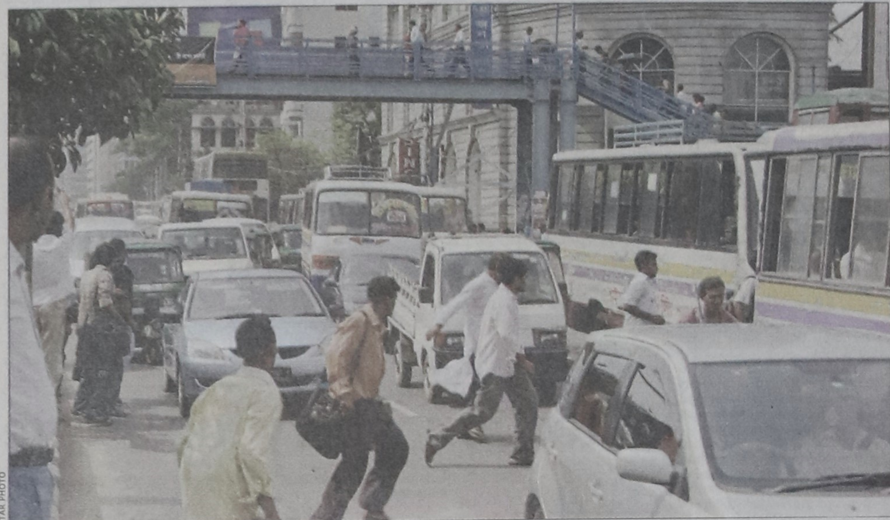
Pedestrians still prefer to risk their lives at the busy intersection at Bangla Motor despite the construction of the much-demanded footbridge.
