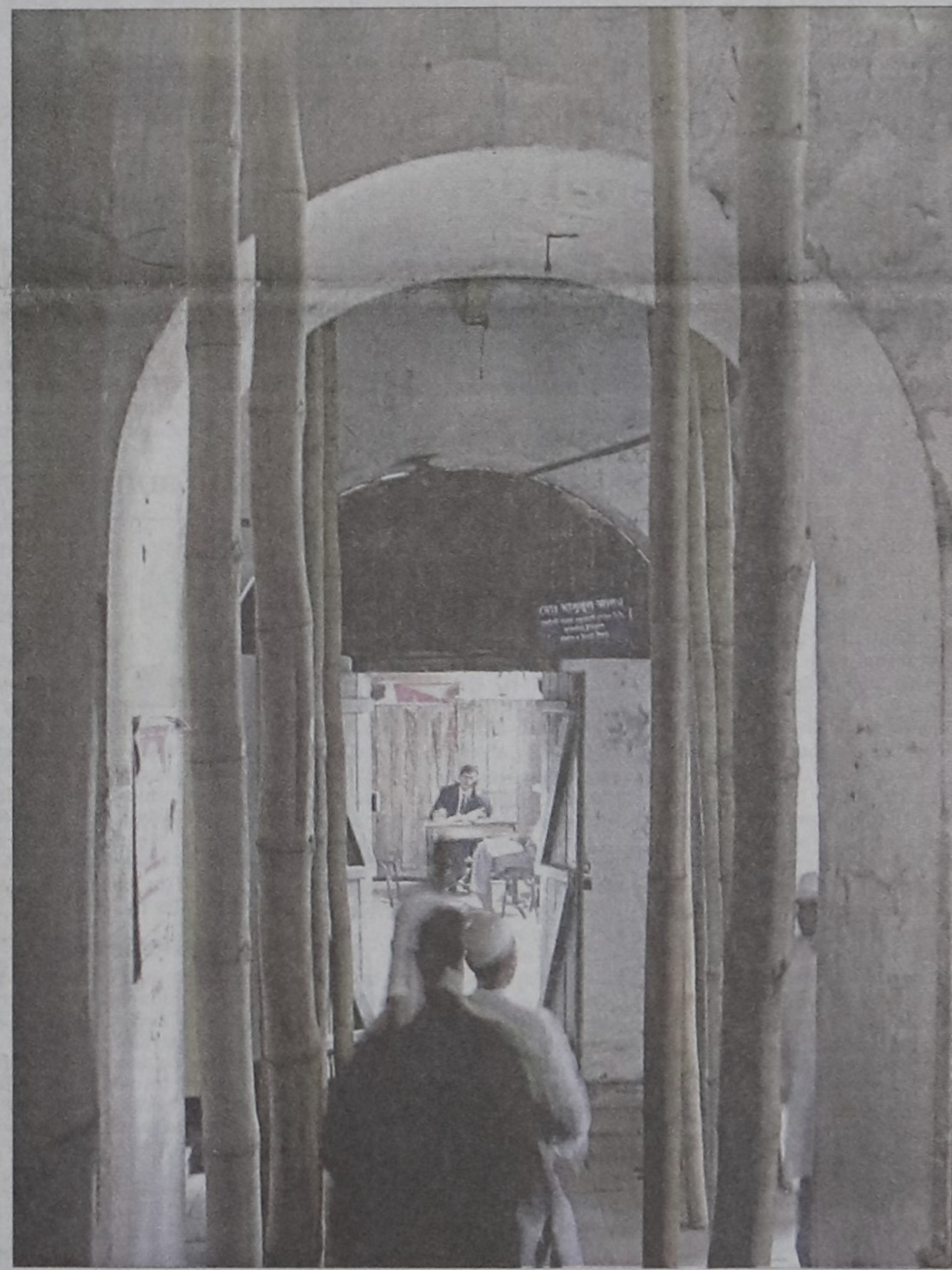
This photo taken yesterday in front of the public prosecutor's office at the Chittagong court building shows bamboos being used for keeping the dilapidated ceiling in place.
