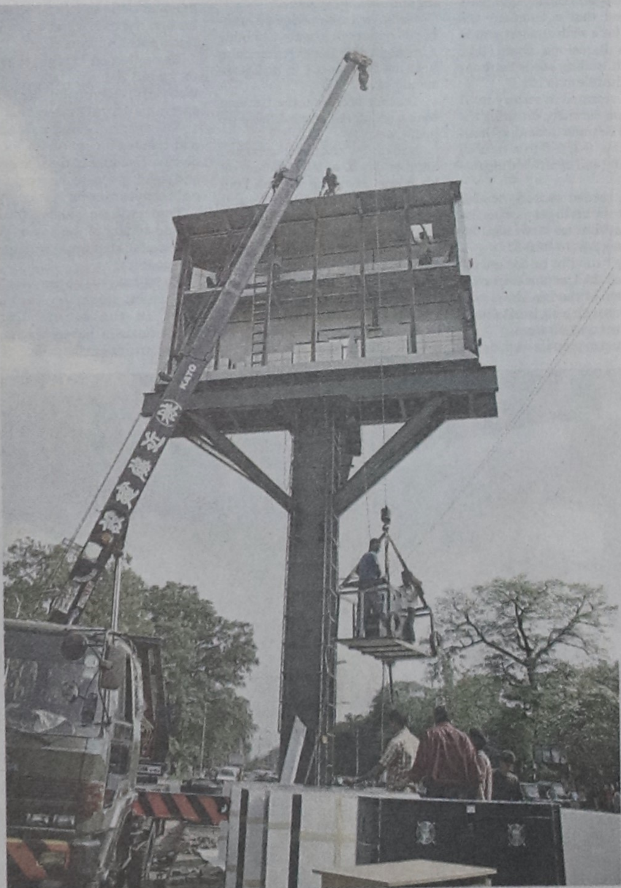
A big television being installed by the Election Commission at Shahbagh to give the voters up-to-date information about preparation for the coming election.
