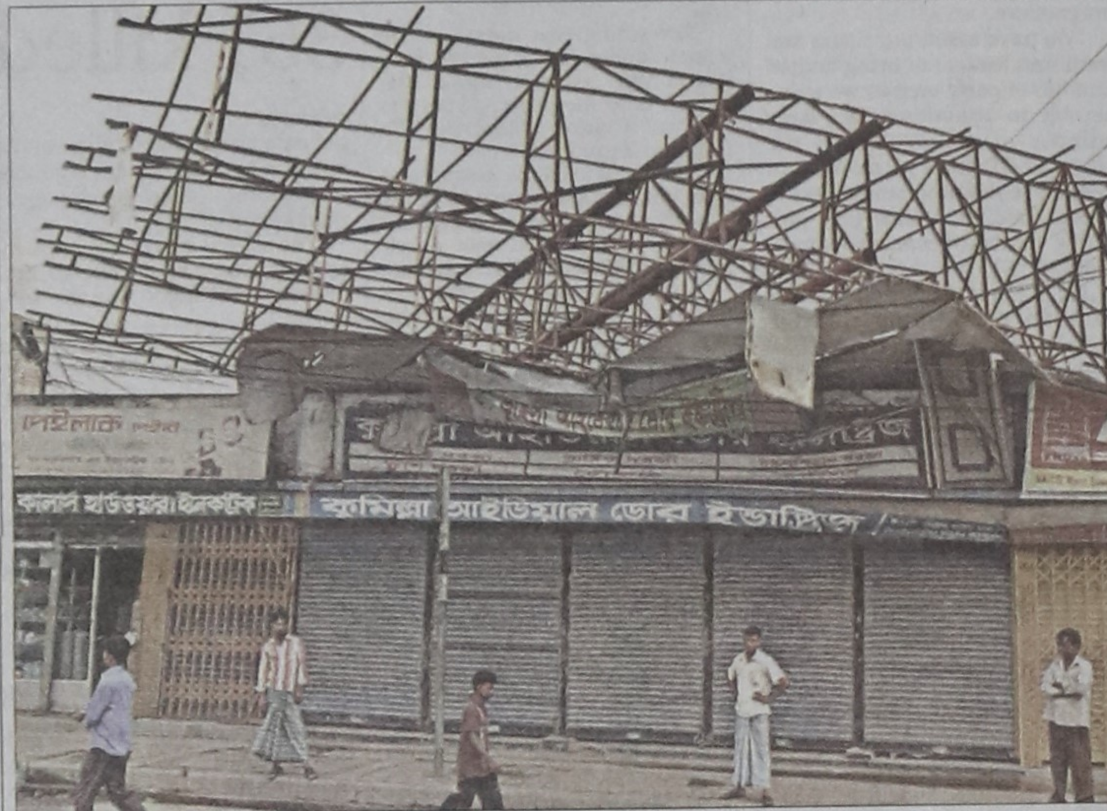
The photo taken yesterday shows a large billboard that collapsed on shops at Merul Badda in the capital during Saturday night's nor'wester.
