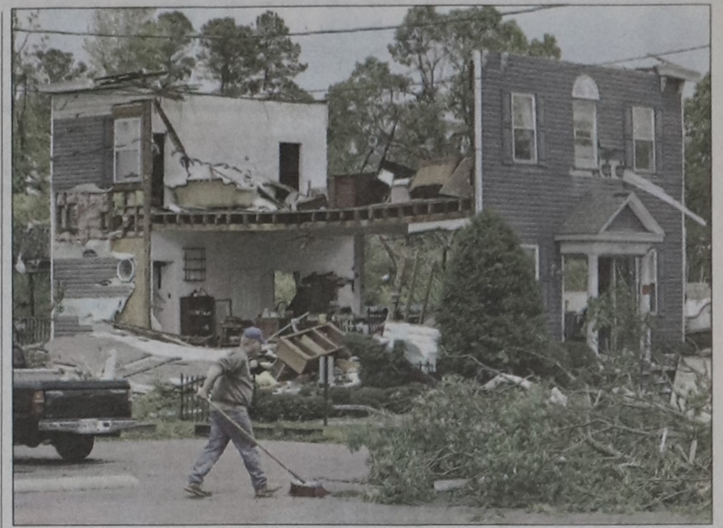
Local resident Jay Thompson cleans up debris in front of the Harmony House Antiques store, which was damaged by a tornado on Tuesday in the Driver area of Suffolk, Virginia. Three Tornadoes touched down in central and southeast-ern Virginia damaging buildings and injuring at least 200 people.
