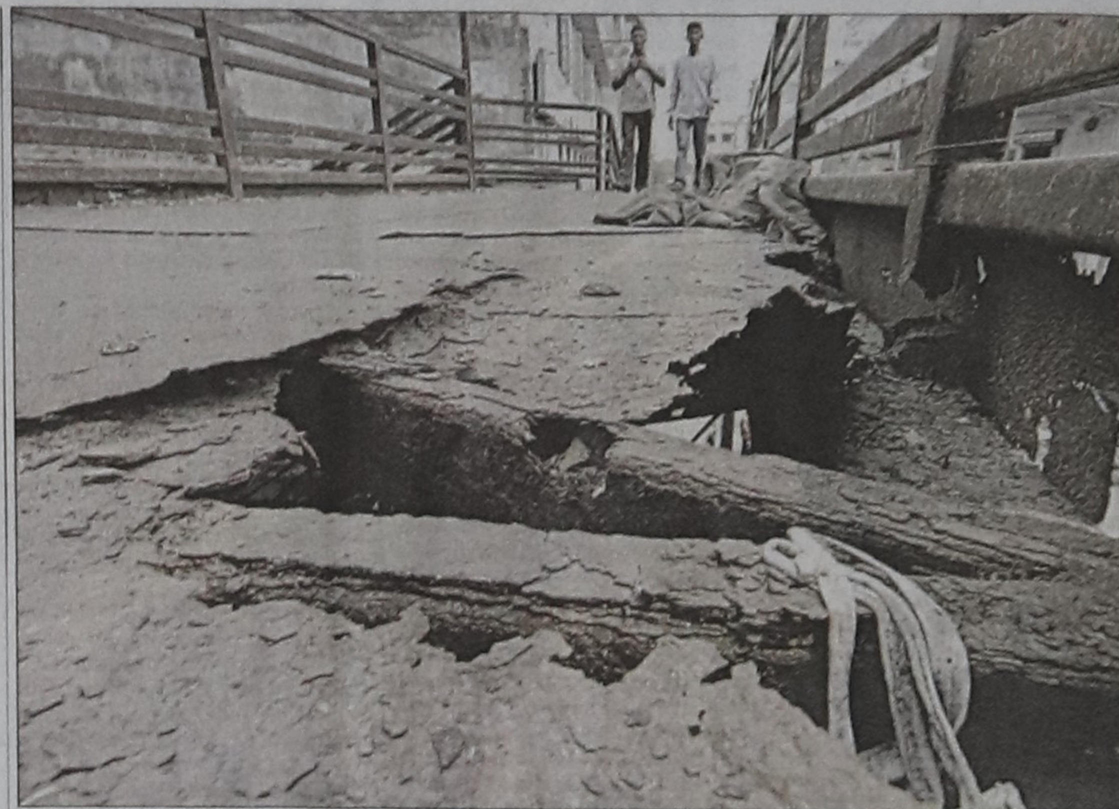
The foot-over bridge at Hatkhola in the capital has developed a large hole for lack of maintenance.
