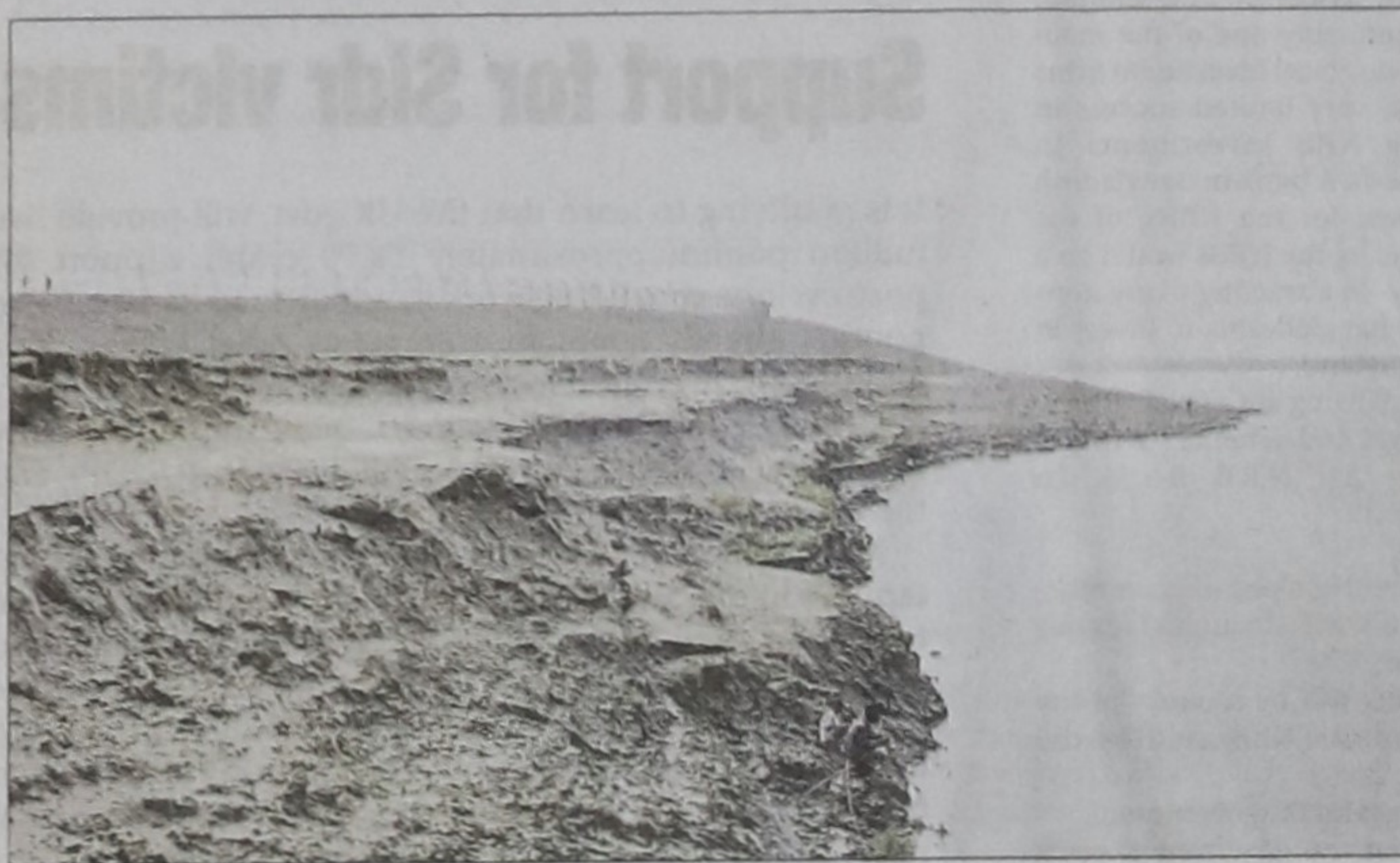
Erosion caused by waves due to rampant plying of sand-laden engine boats threatens the east side guide embankment of Jamuna Bridge, left, boats wait for loading sand at a river channel.
