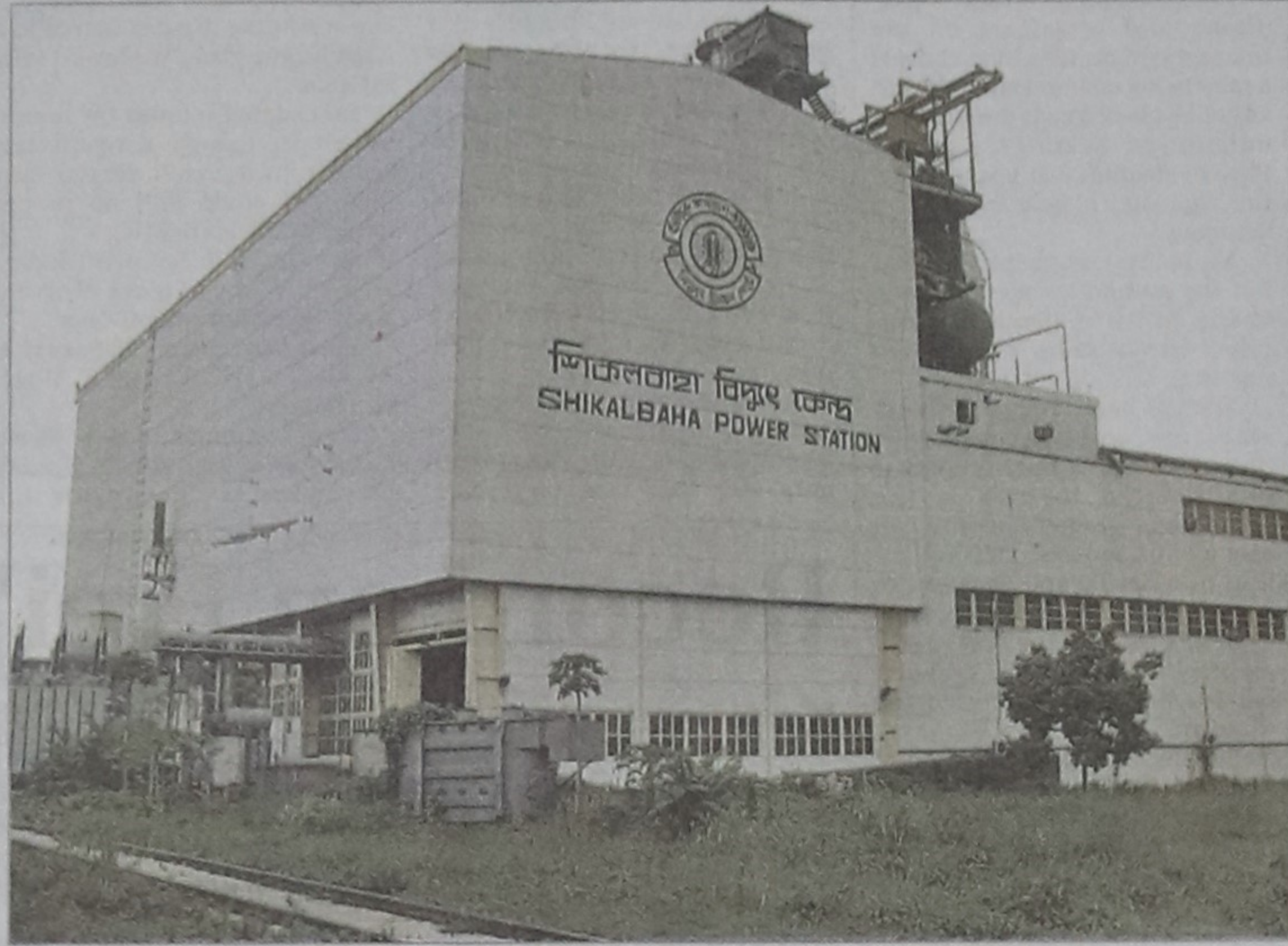
Shikalbaha Power Station.
