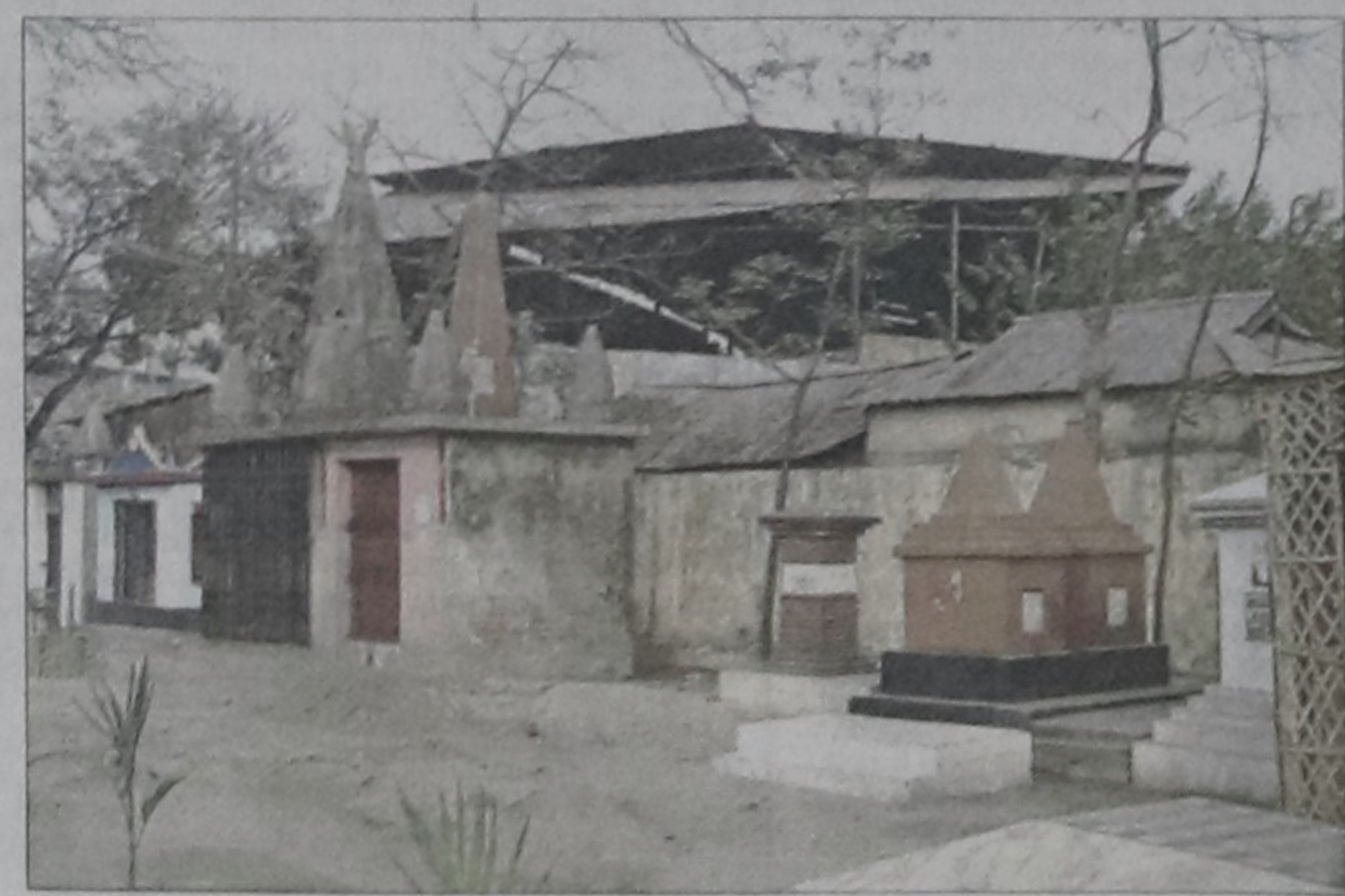
Tin roof of a re-rolling mill overlooks the burial ground, allegedly encroaching a part of the Postogola cremation ground.
