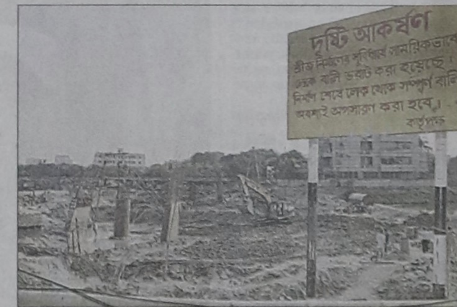
The Gulshan-Banani Bridge project site.
