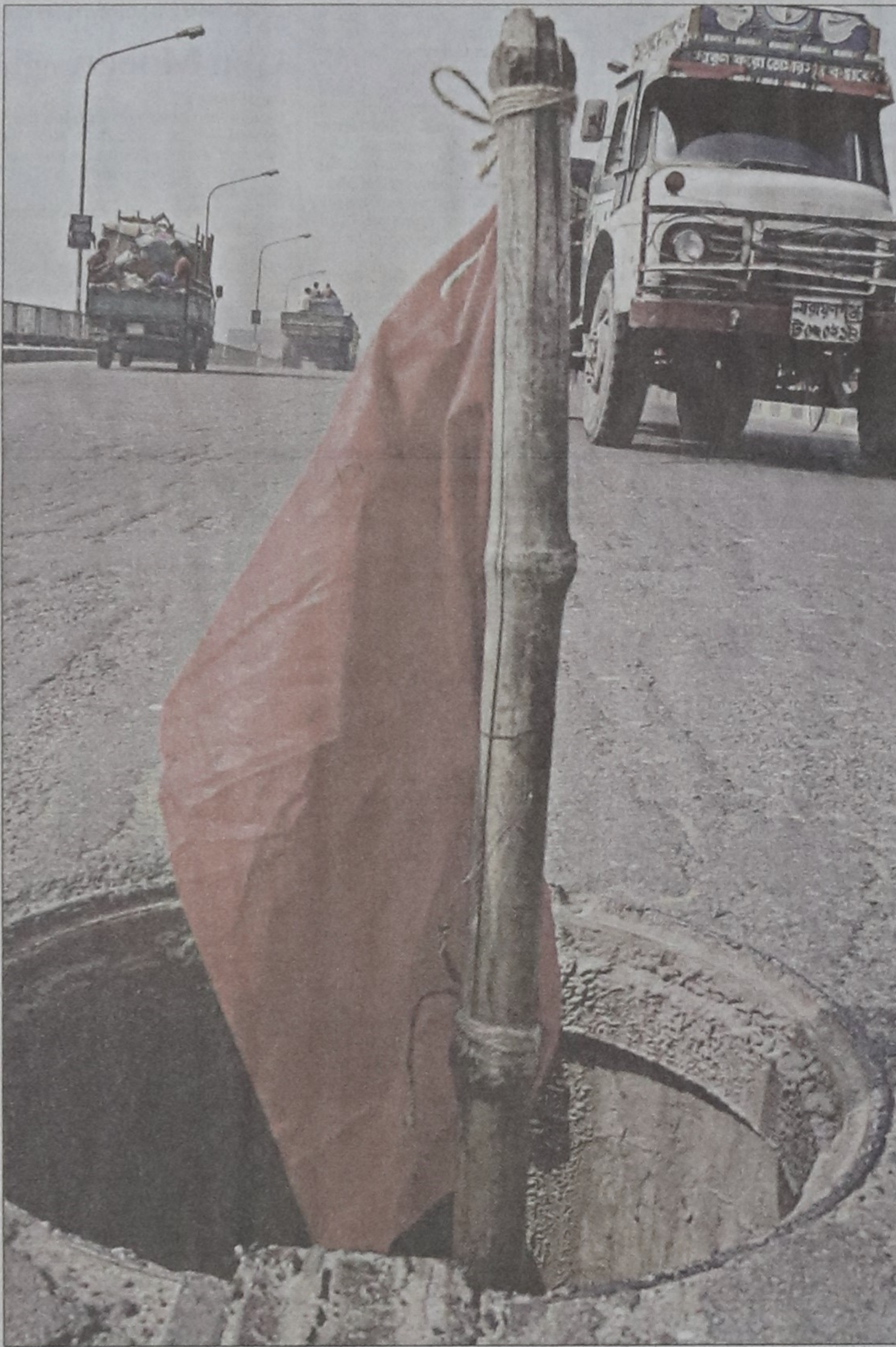
A red cloth tied to a bamboo pole jutting out of a lidless service manhole on Bangladesh-China Friendship Bridge at Postogola as a warning to approaching vehicles.
