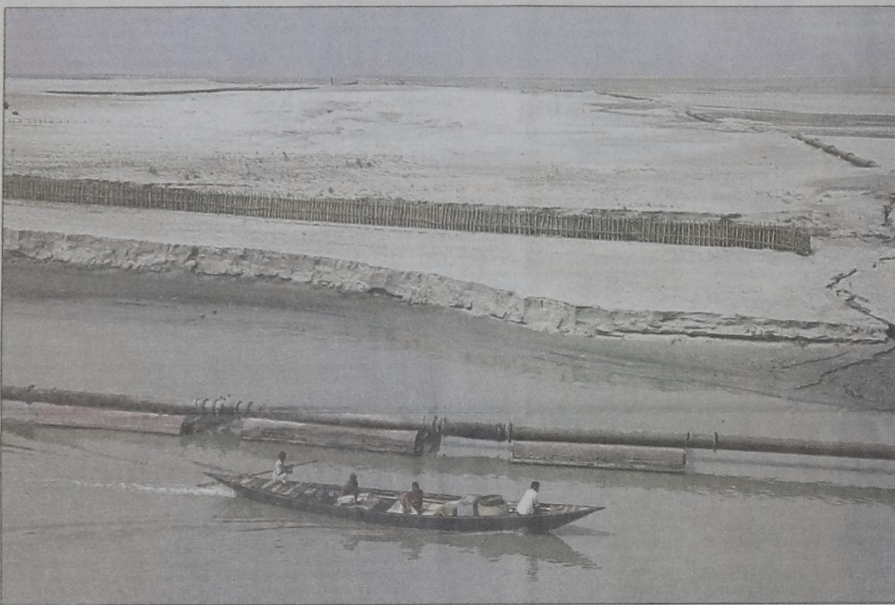
A narrow channel is dredged through a char in the Padma near Paturia to keep the Paturia-Doulatdia ferry service alive.
