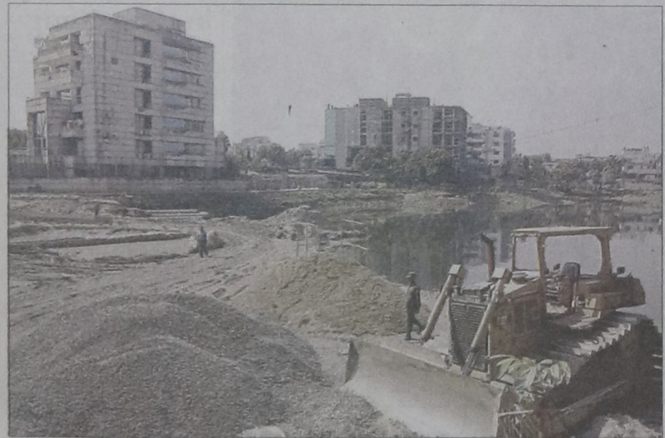
Star file photo of construction of the bridge over Gulshan Lake.
