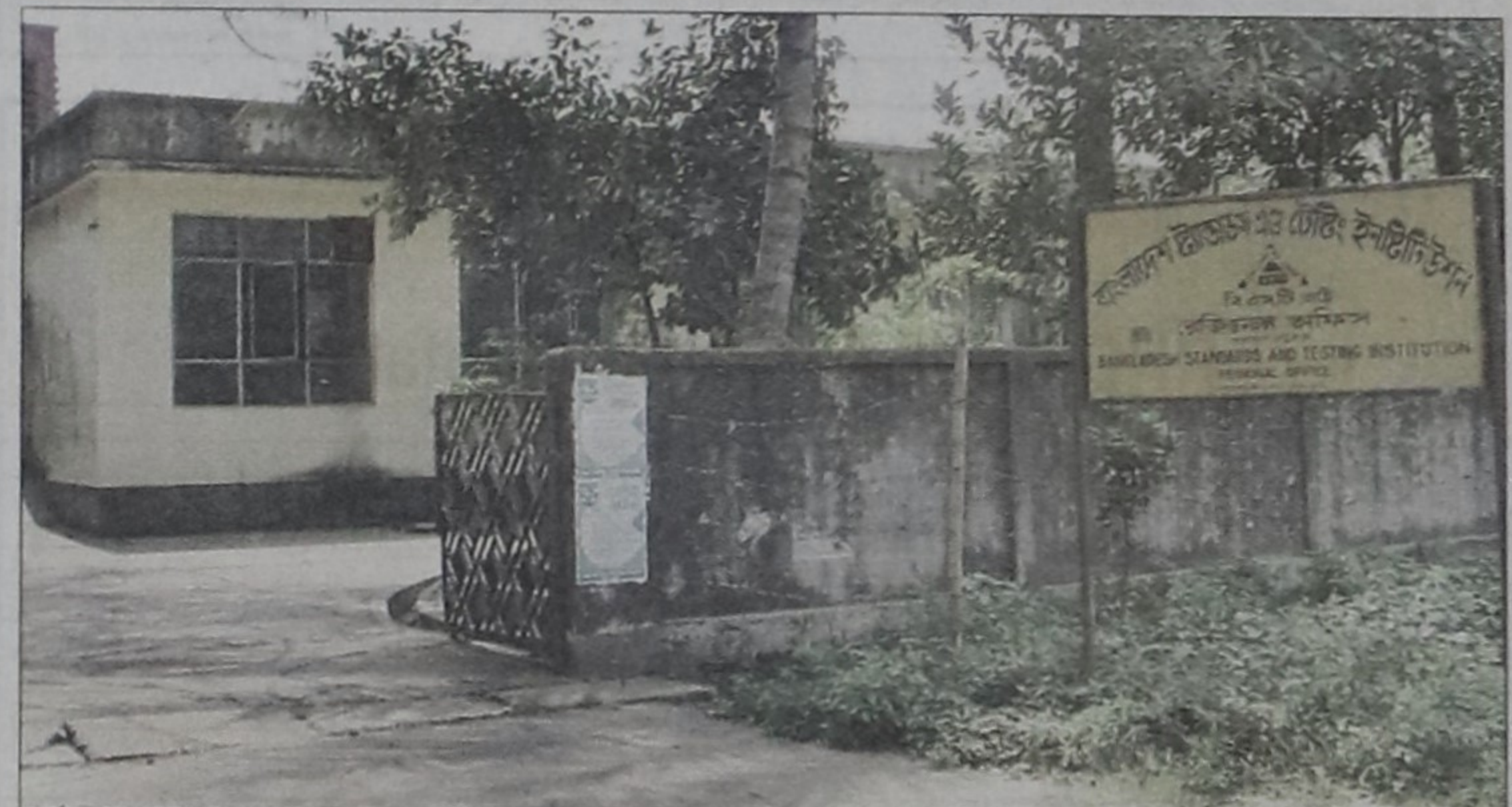
Bangladesh Standards and Testing Institution (BSTI) Chittagong regional office at Agrabad.
