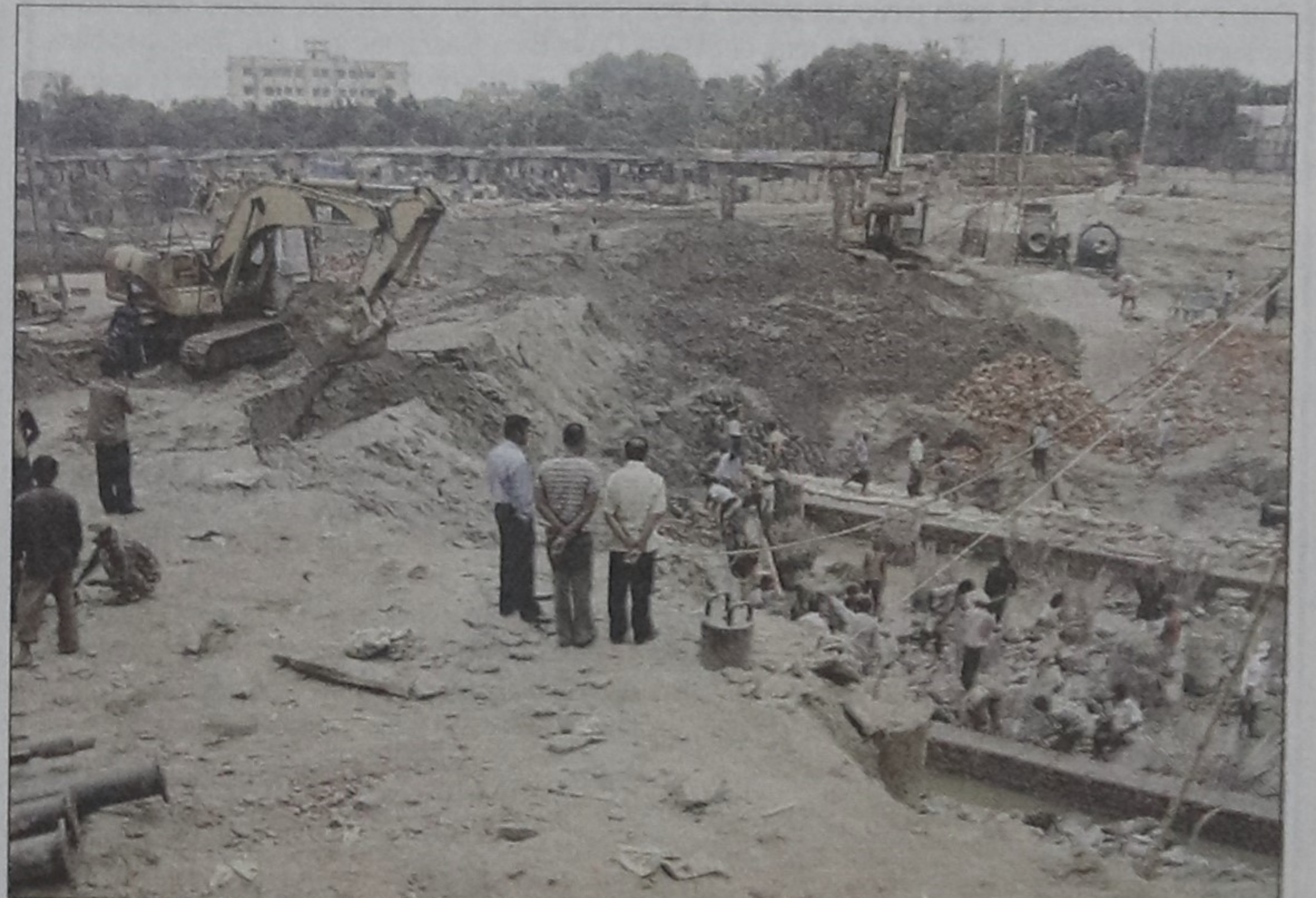
Work on the Gulshan-Banani Bridge in progress.
