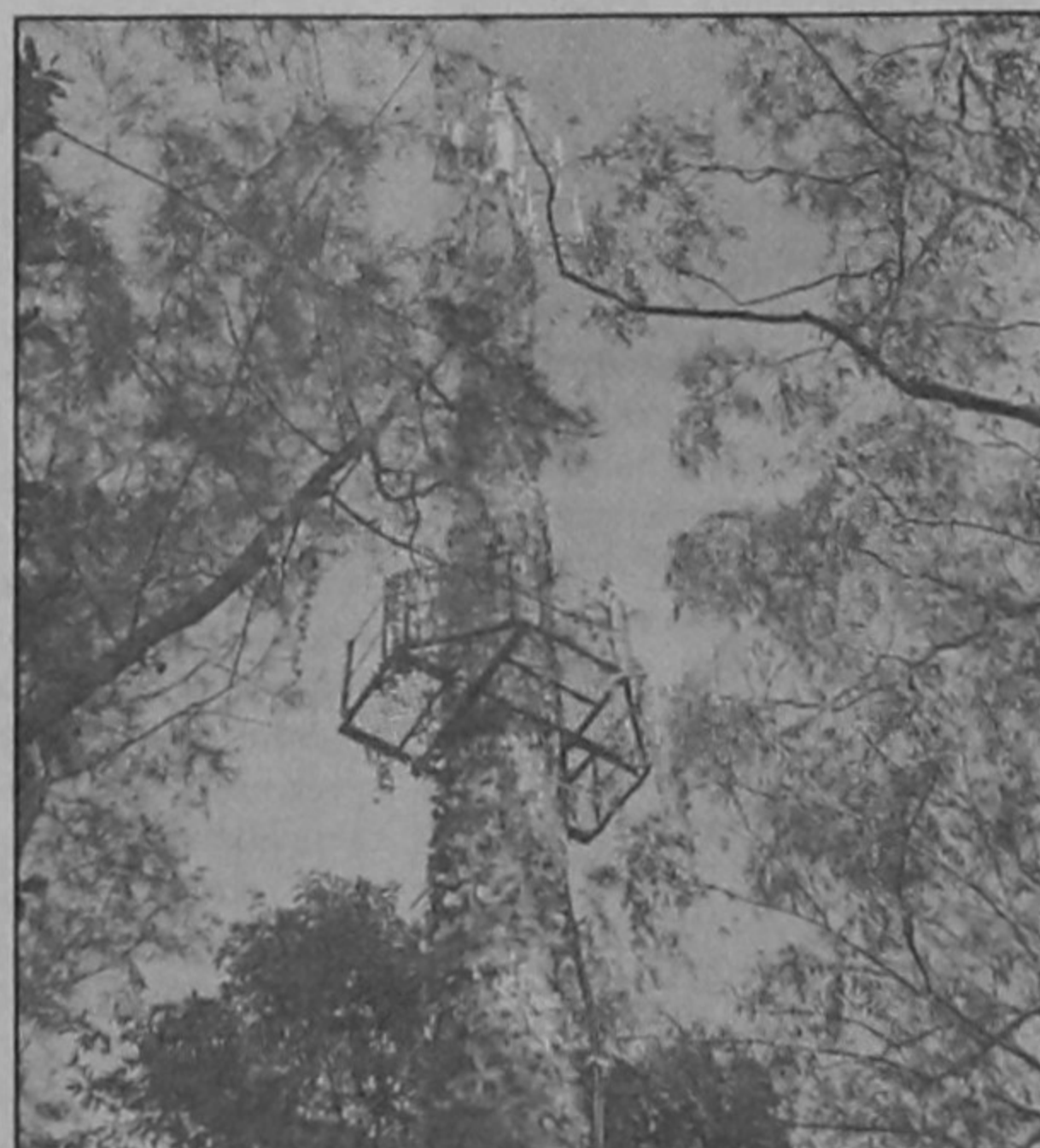
A monopole base station erected by Grameenphone in Dhaka. The pole has been camouflaged to look like a tree trunk, although work still needs to be done to hide the equipment at the top of the tower.
