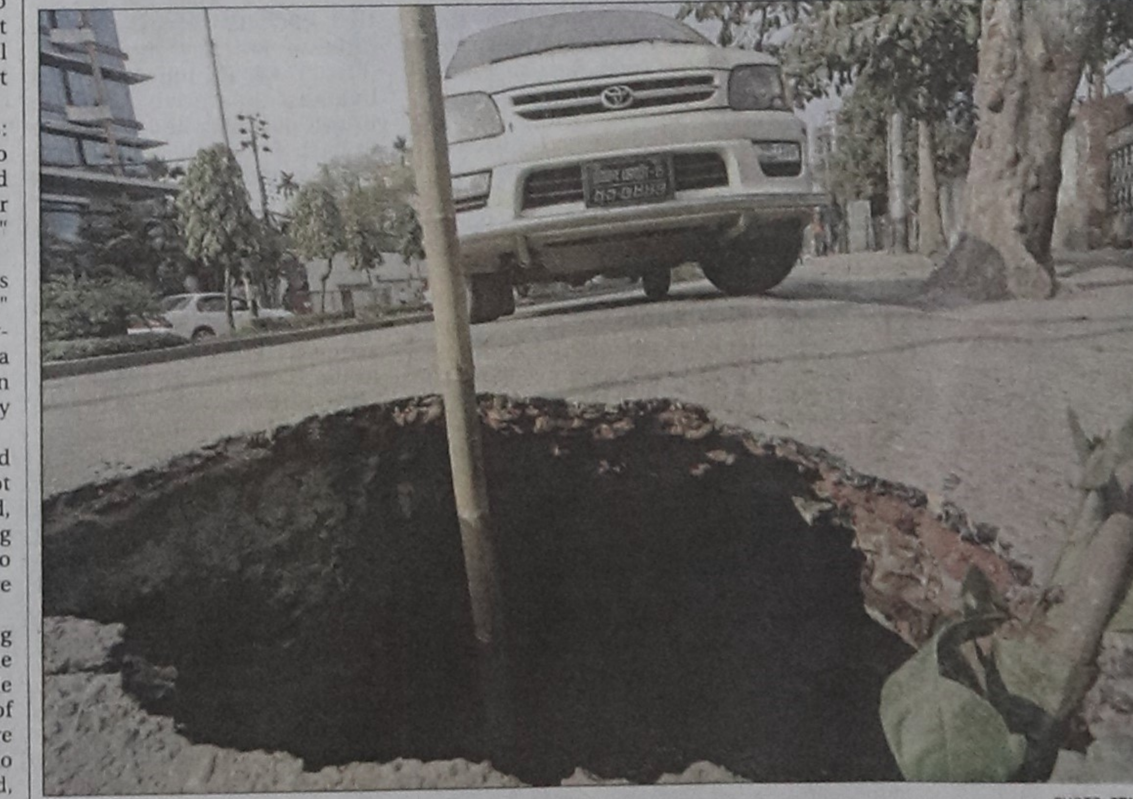
The photo taken yesterday shows a bamboo put by locals in the gaping hole on Road-140 at Gulshan in the capital. The bamboo is the only sign warning vehicles of the danger.
