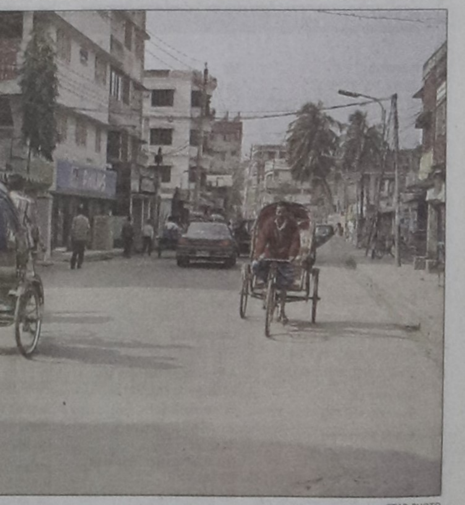
The Basabo-Nandipara Road narrowed down (1) and widened up (2) at different points discouraging introduction of major transport system in the area.
