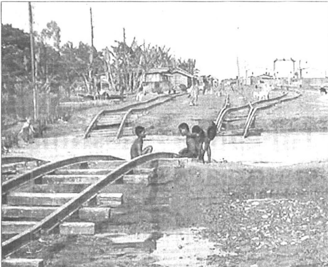
Flood-ravaged railway tracks on Trimohony-Balashi section near Balashi rail yard in Gaibandha. The repair work is yet to start.
