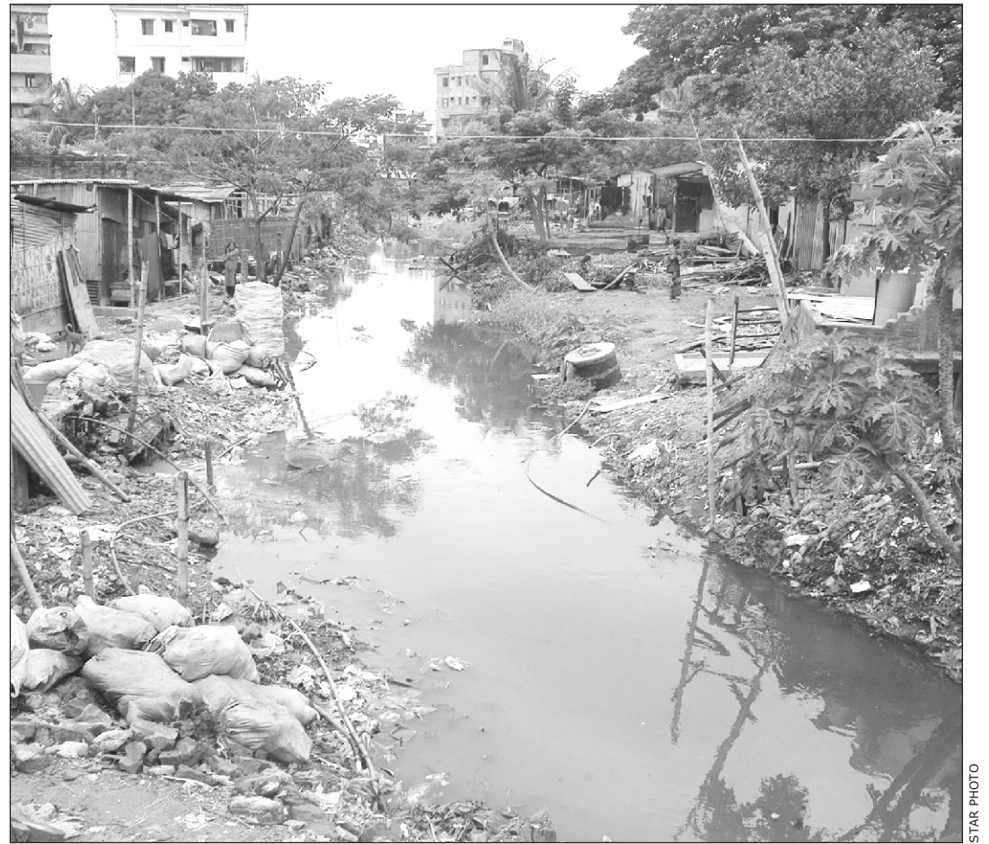
Ibrahimpur canal: Badly in need of urgent 'rescue'.
