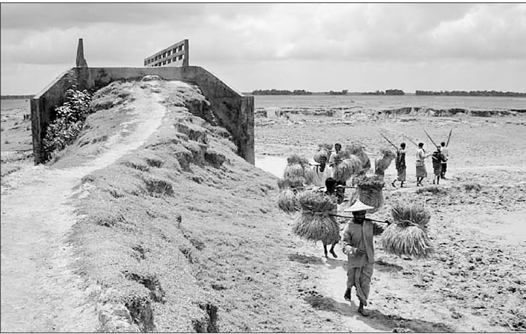
PHOTO: RAJAT KANTI GOSWAMI A newly constructed culvert on Doldoli canal of Kamarchalk union in Rajnagar upazila, Moulvibazar, has become useless due to incomplete earth work on the approach towards the Palpur-Dholai Ferryghat Road. It was an example of development in the area during immediate past BNP led 4-party Alliance rule.
