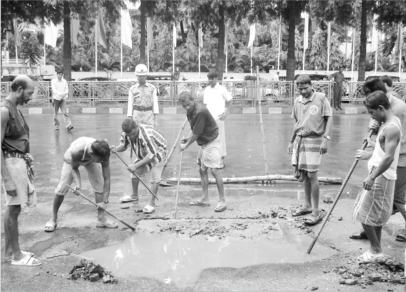
DCC workers yesterday ripped open the manhole near the entrance of Karwan Bazar in front of the hotel Sonargaon. The workers said that the same manhole has been repaired 25 times over the course of last 3 years, costing the DCC lakhs of taka, without permanently solving the problem.
