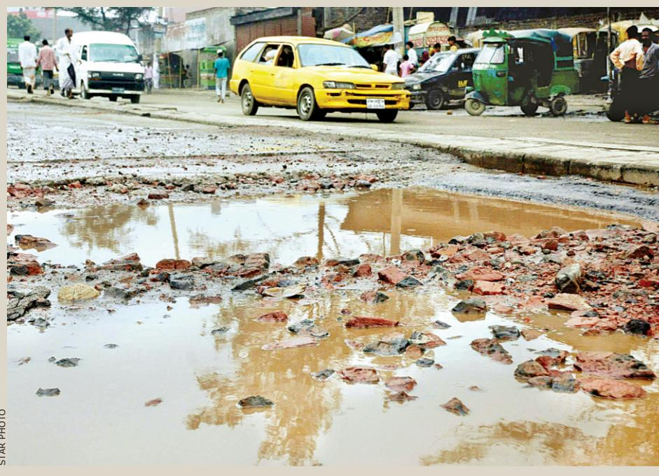
Parts of the main road at Hasnabad near the first Buriganga bridge is almost unusable. The road gets flooded with slight rains when traffic jam builds up as vehicles slow down to cross the dilapidated area.
