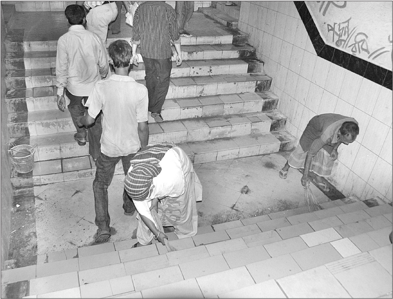
Following a story published in Star City on May 28, 2007, the Dhaka City Corporation (DCC) finally took initiatives to repair the shabby underpass in the Sonargaon intersection of the city. Workers were seen repairing the broken stairways by filling in the cracks with marble slabs while sweepers were cleaning the scattered debris littering around the whole place. The authorities have also installed new tube lights to improve lighting facilities in the underpass. However, the overhead sewerage pipes are yet to be repaired while the graffiti that stretches across the wall needs to be removed.
