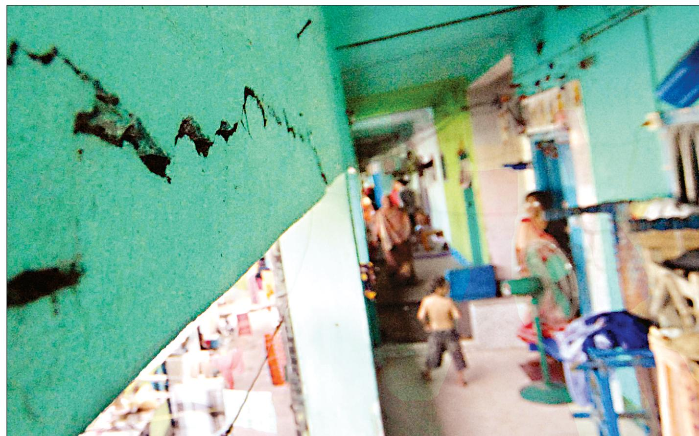
Poor quality building materials caused structural failure and cracks in the walls and columns of the newly built six-storey building in Dayaganj sweeper colony in Sutrapur.
