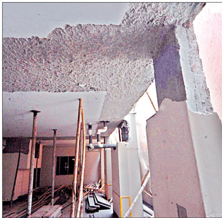
An inside view of an apartment building, left, of Amin Mohammad Foundation that developed cracks forcing its residents to evacuate. The outer view, right, of the building at Dhanmondi in the capital.
