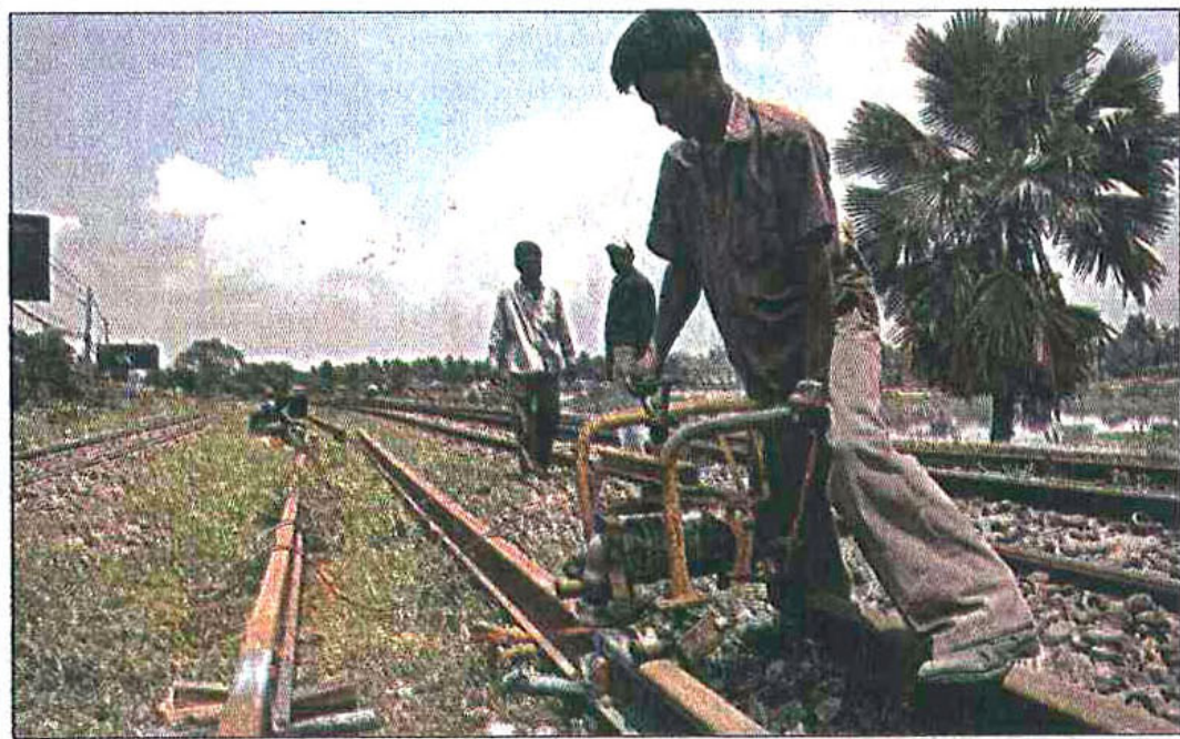
Workers of Bangladesh Railway turn the metre-gauge lines into dual-gauge at Khilkhet in the capital to facilitate Dhaka-Kolkata direct train service which is likely to begin from August.
