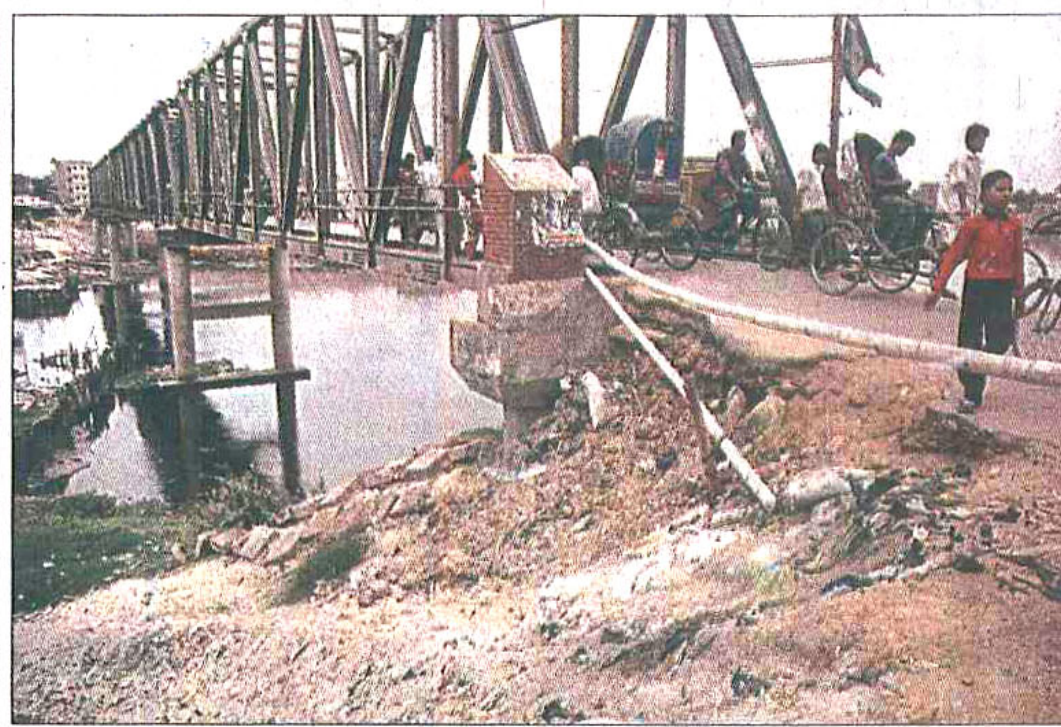
This steel bridge connecting the capital with suburb on Kamrangirchar on the other side of the Buriganga River is now in a vulnerable condition as the ground holding the pillars has loosened.
