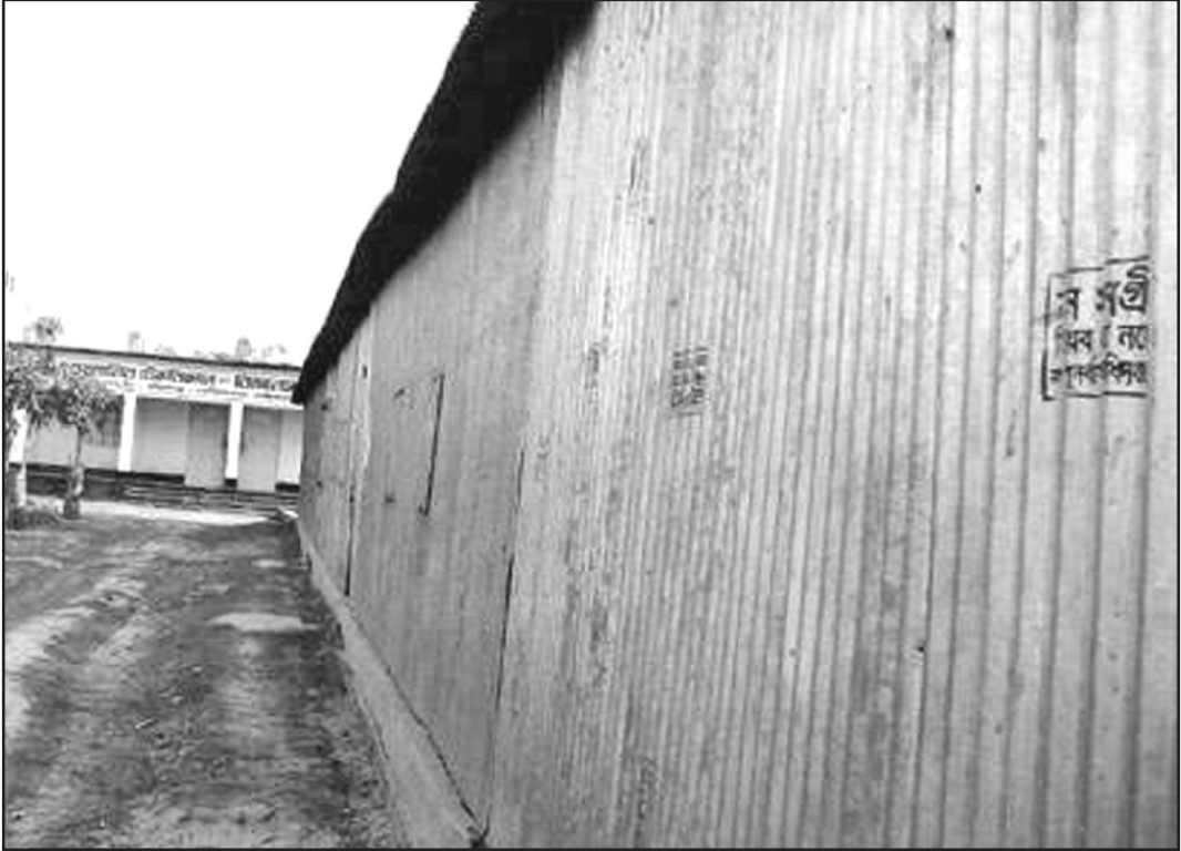
Relief CI sheets used in MAMuttalib Technical and BM College in Mohimaganj in Gaibandha are still intact.
