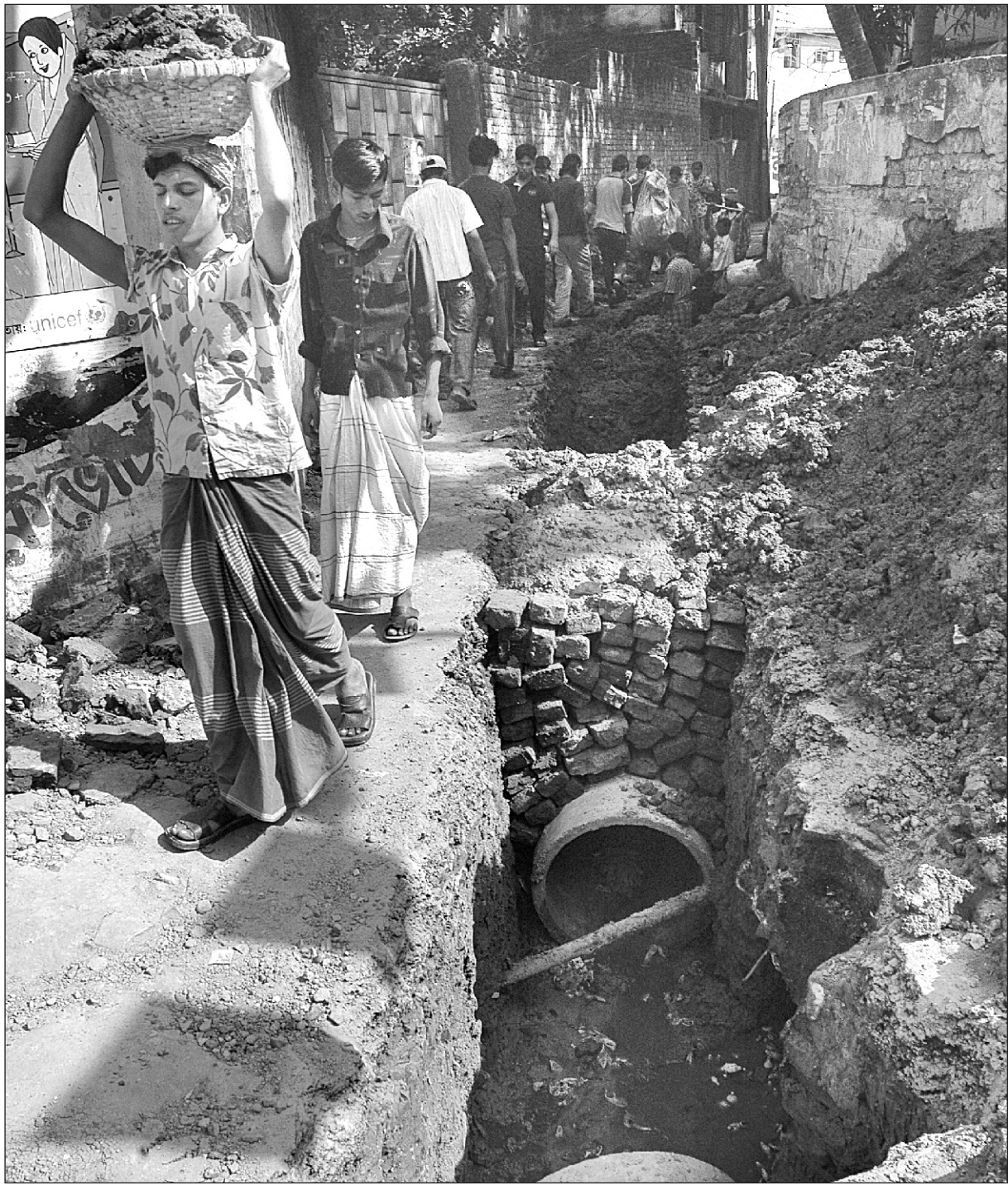
For the last few days this road, in front of Segunbagicha School, is dug up for the installation of sewerage line. The line which should have been implanted before paving the road shows a glaring
