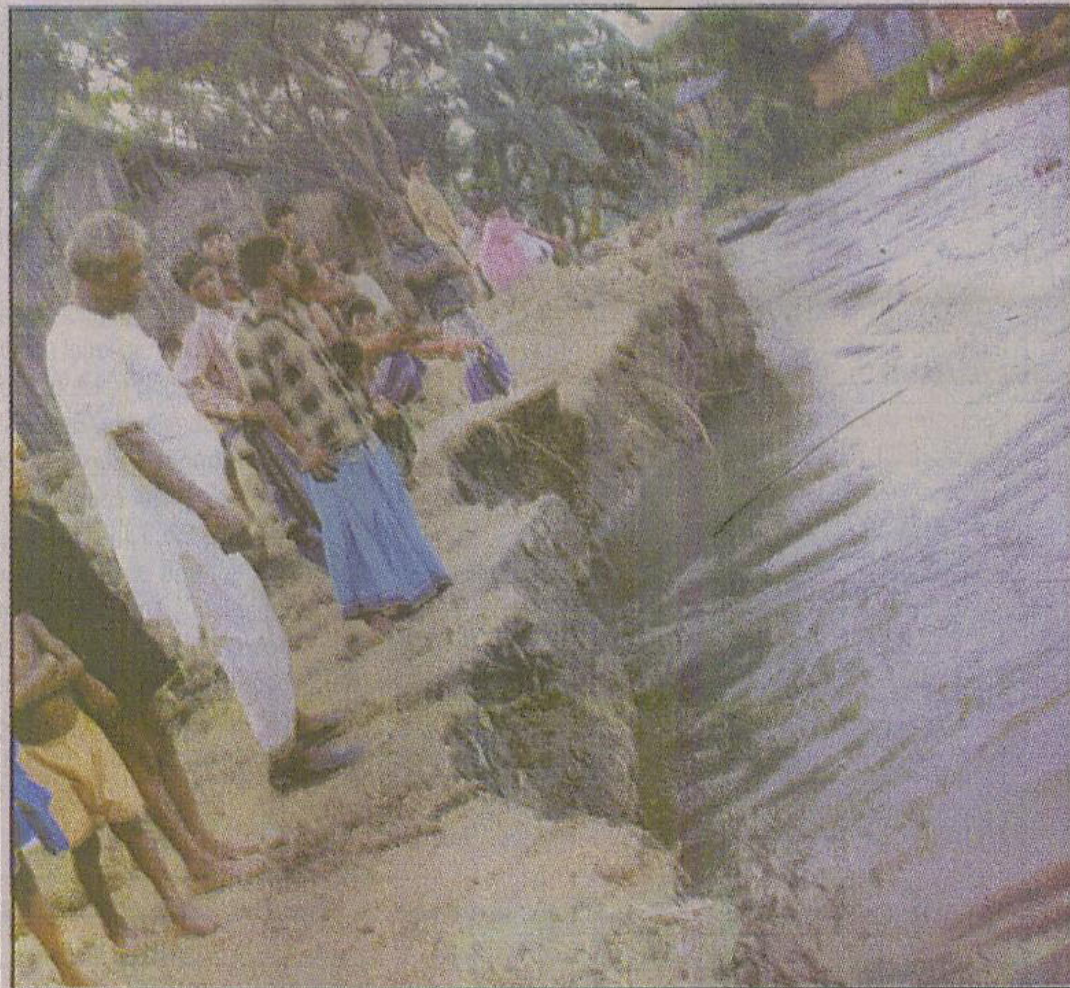
PHOTO: STAR The Kalni river devoured at least 50 homesteads in Derai upazila in Sunamganj district in about a week. Panicked villagers watching the river erosion to decide when to shift their houses.
