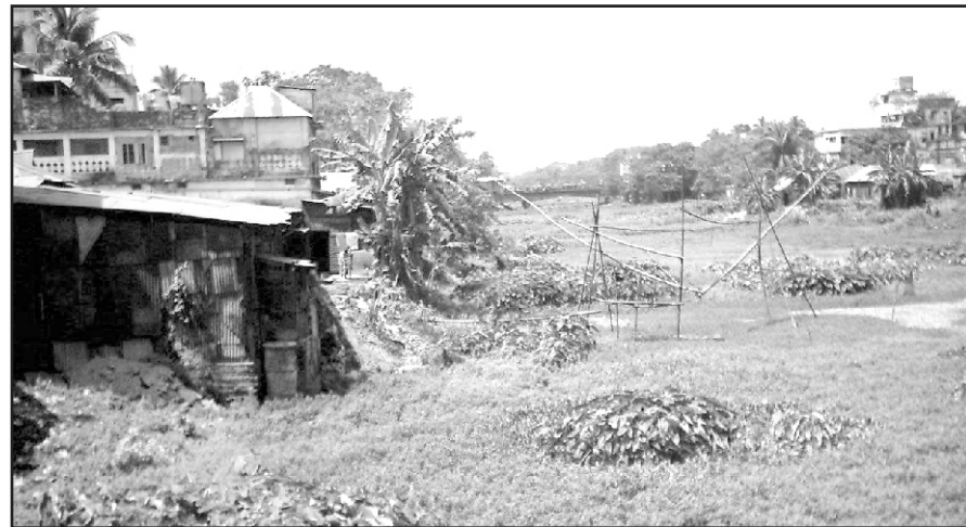
Houses being built on silted up Naroshonda river (left) and makeshift shops and structures on a bridge on the rivers in Kishoreganj town.
