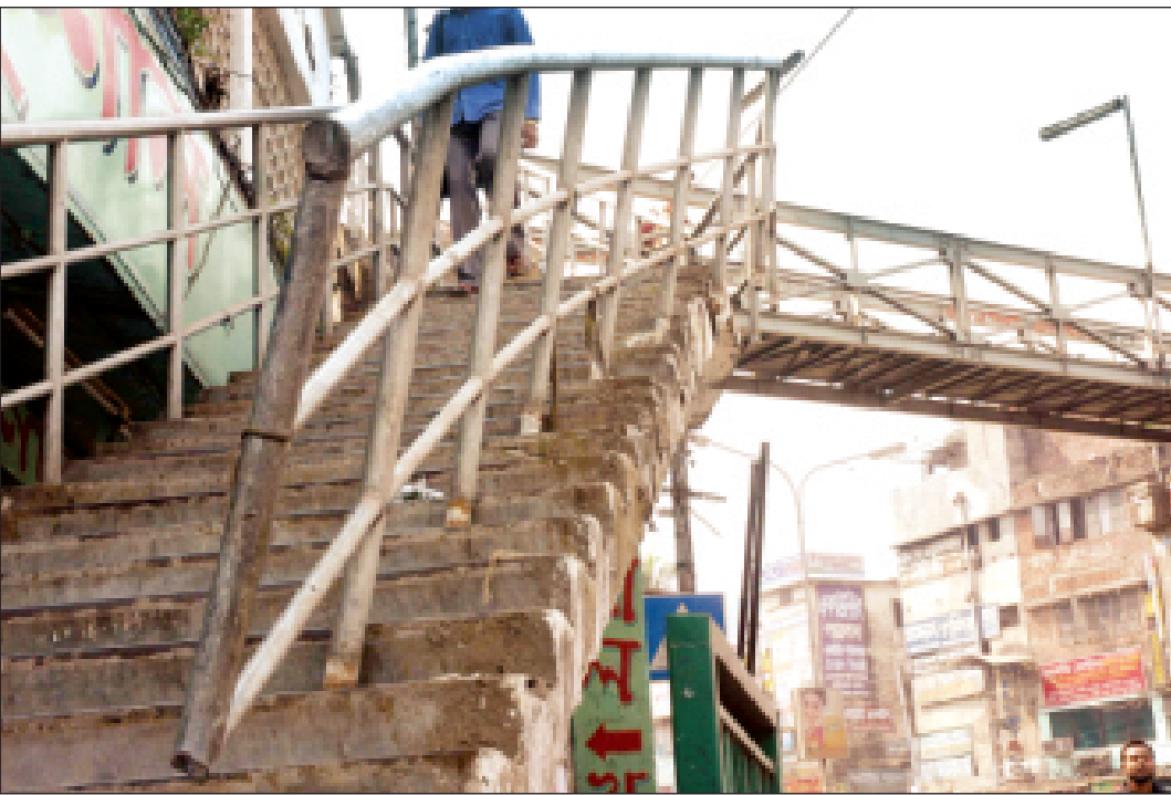
A displaced railing on the stairs of the foot over-bridge at Science Laboratory intersection in the capital remains uncared for, leaving pedestrians in danger for over a week.
