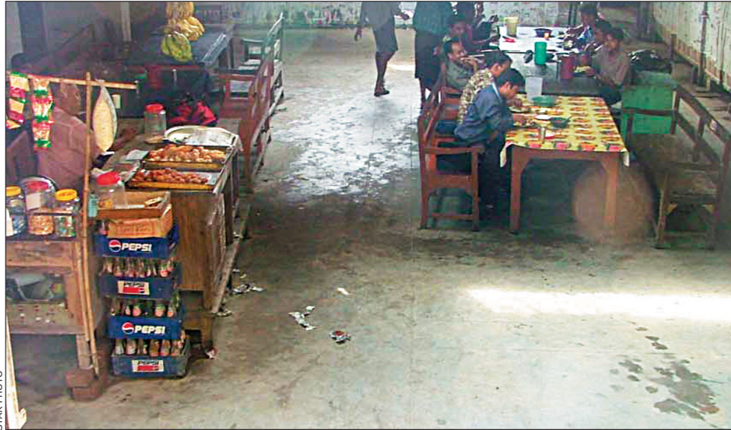
The dilapidated cafeteria at the Arts Faculty Building basement at Chittagong University.
