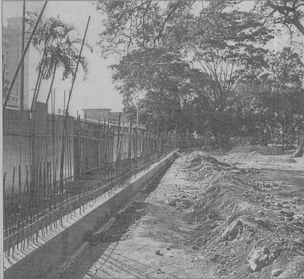
Renovations and beautification are underway at the Osmani Uddyan.
