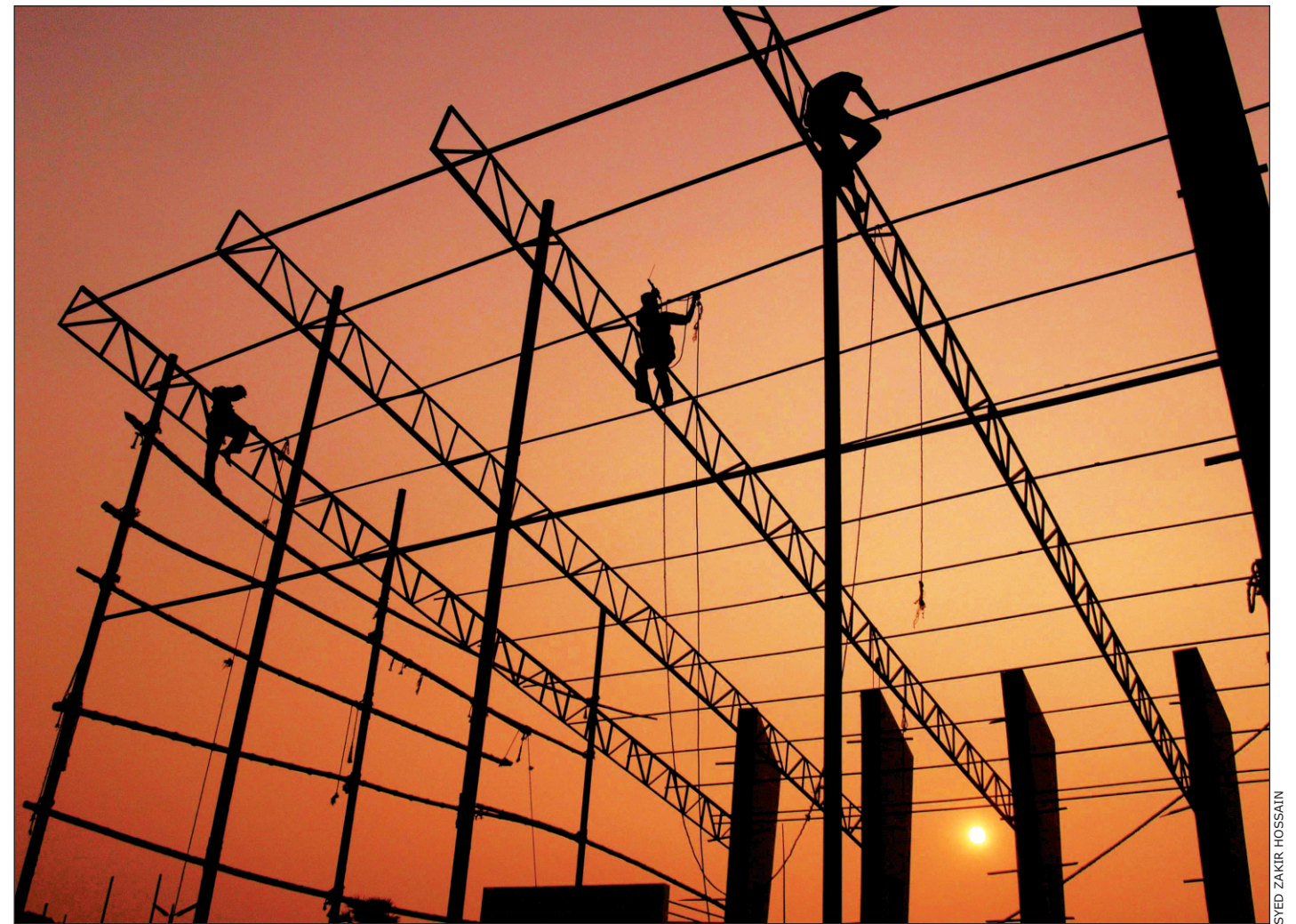
Work on a pavilion goes on at the DITF venue.
