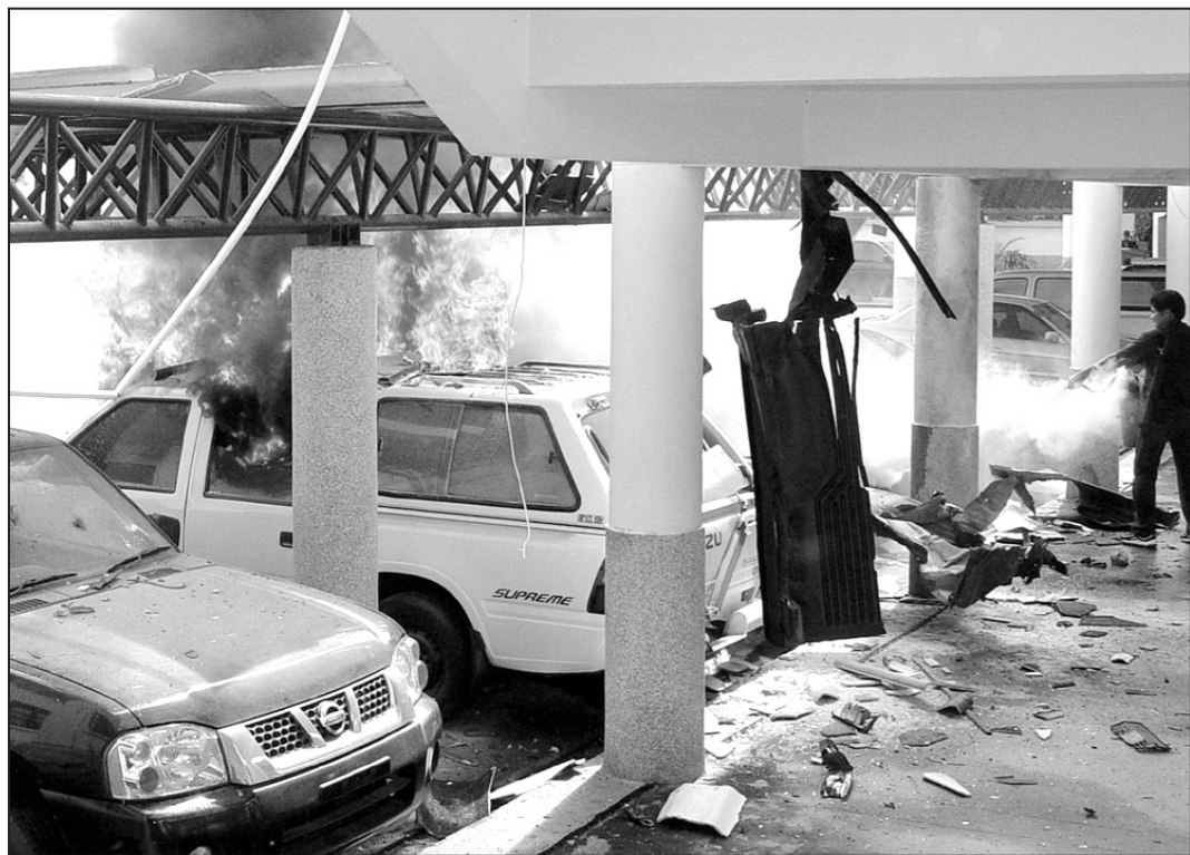
A Thai employee tries to extinguish fire following a bomb blast in the parking area of a provincial government building in Thailand's violence raged southern Yala province yesterday. Two bombs went off at two different government buildings in Yala after a night of deadly gun battles, as Prime Minister Thaksin Shinawatra insists security forces are making gains in their fight against Islamic dissidents.
