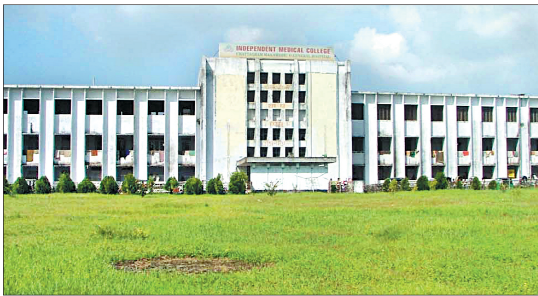
The Maa-Shishu O General Hospital building complex at Agrabad.
