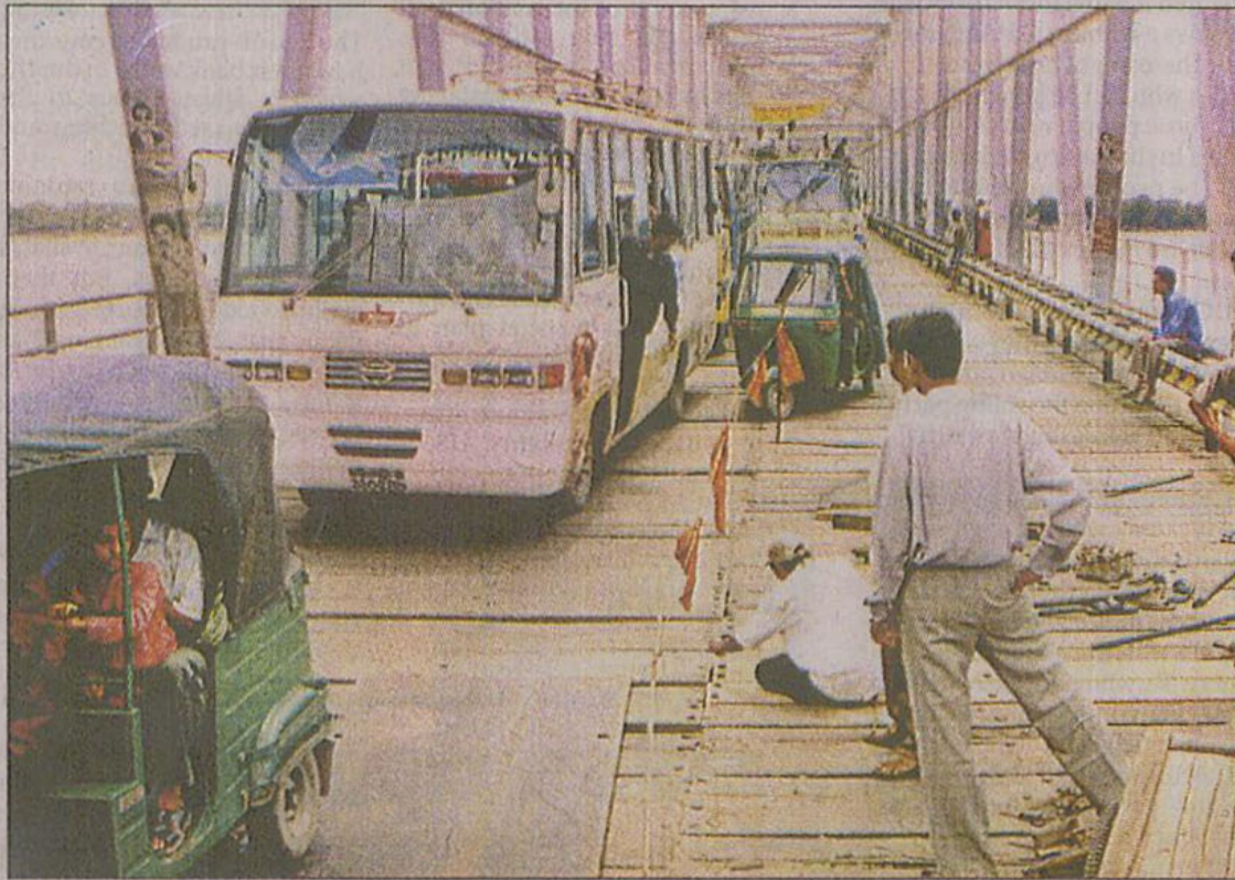
(Right) A truck on Saturday night gets its wheels stuck in the broken wooden deck while trying to pass illegally through the Karnaphuli Shah Amanat Bridge. (Left) For lack of the wood required for repair work, the deck is fixed with the previously leftover or rejected wood..
