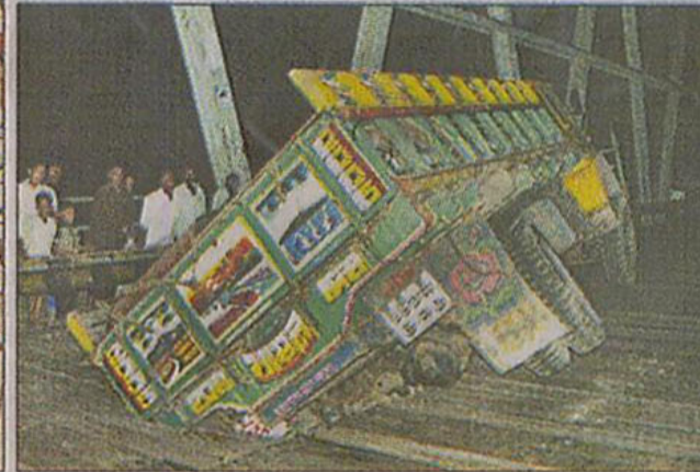
(Right) A truck on Saturday night gets its wheels stuck in the broken wooden deck while trying to pass illegally through the Karnaphuli Shah Amanat Bridge. (Left) For lack of the wood required for repair work, the deck is fixed with the previously leftover or rejected wood..
