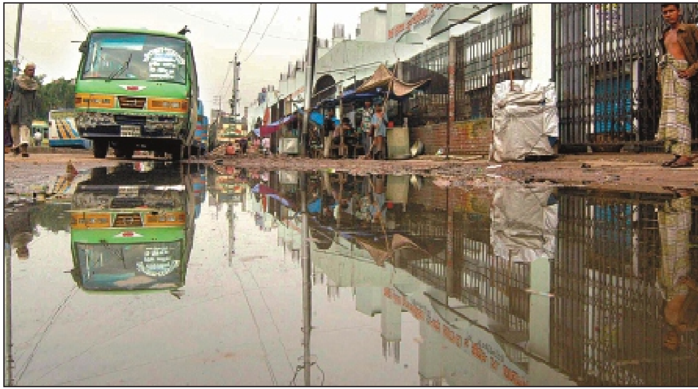
Water remains stagnant on the road adjacent to the Fulbaria Hawkers' Market for hours even after little rainfall due to poor drainage system.
