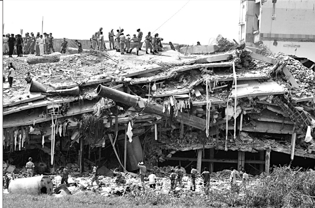
Spectrum building collapsed due to faulty construction
