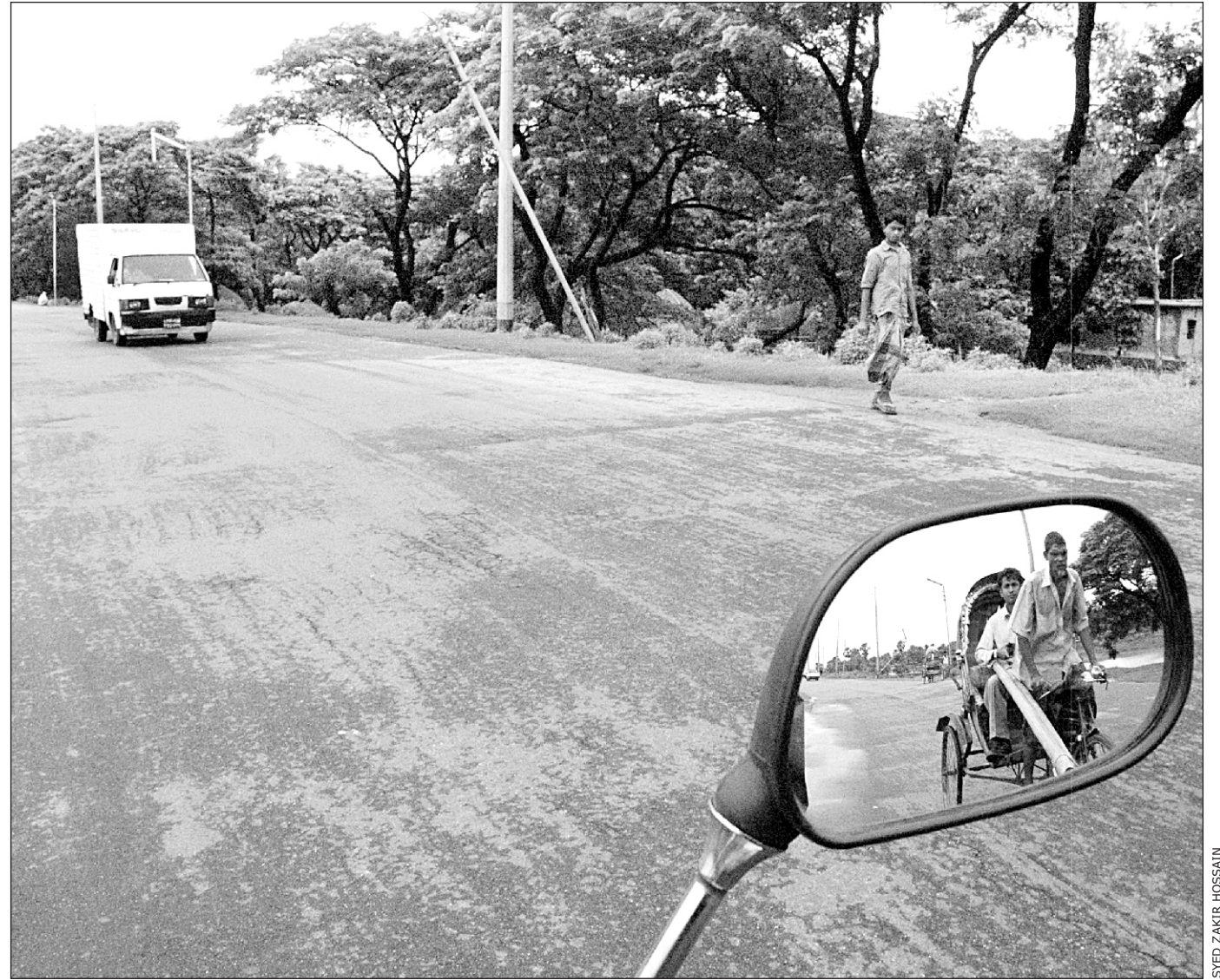
The Western Embankment Road stretching from the Buriganga bridge to Ashulia is earmarked for widening.
