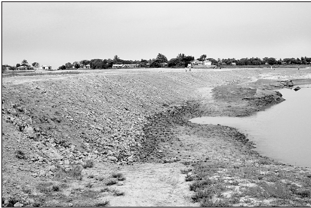
A portion of the 33 km dam built by UNDP in Kishoreganj
