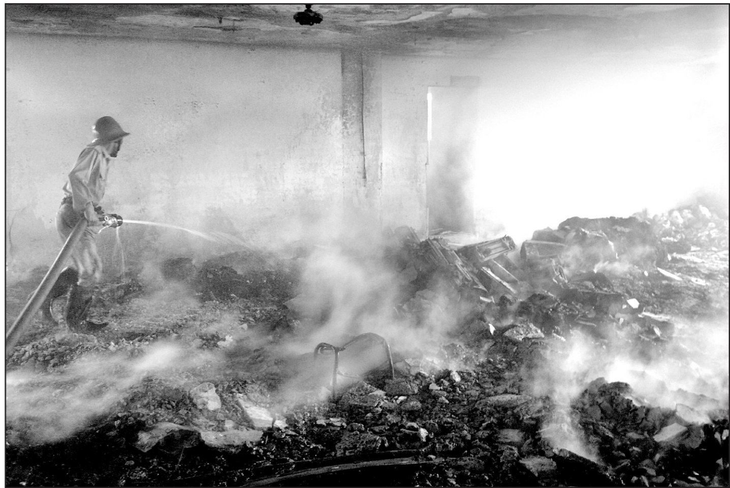
A six-storey export-oriented Biswas Textile and Garments Factory in Savar was damaged in a fire yesterday.
