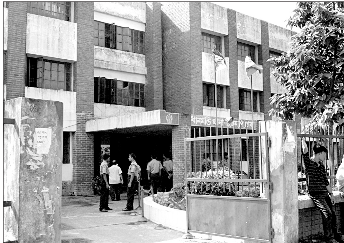
The Dhanmondi Police Station which will be divided into two sections.
