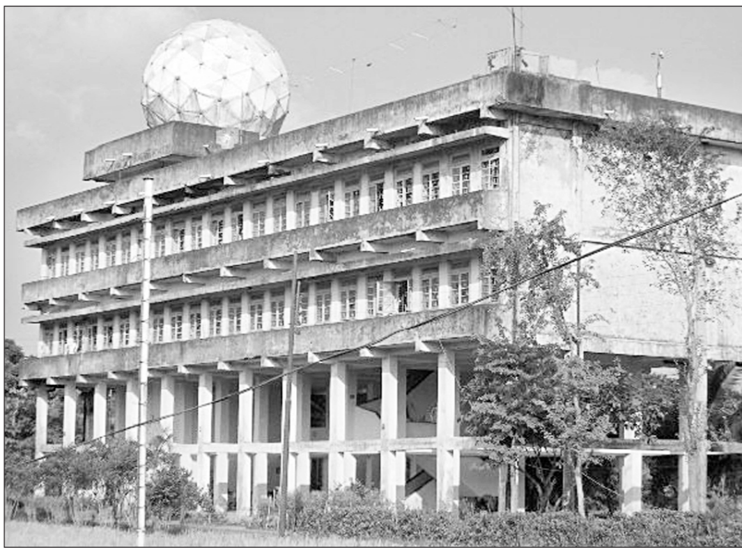
The massive but mute Kalapara radar station.
