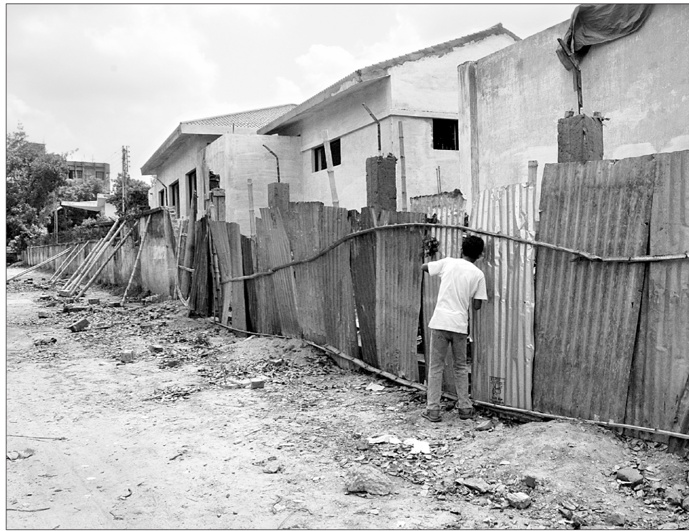
Tin fences have come up along the boundary of the Airforce Officers' Mess at Shaheenbagh instead of solid brick walls.
