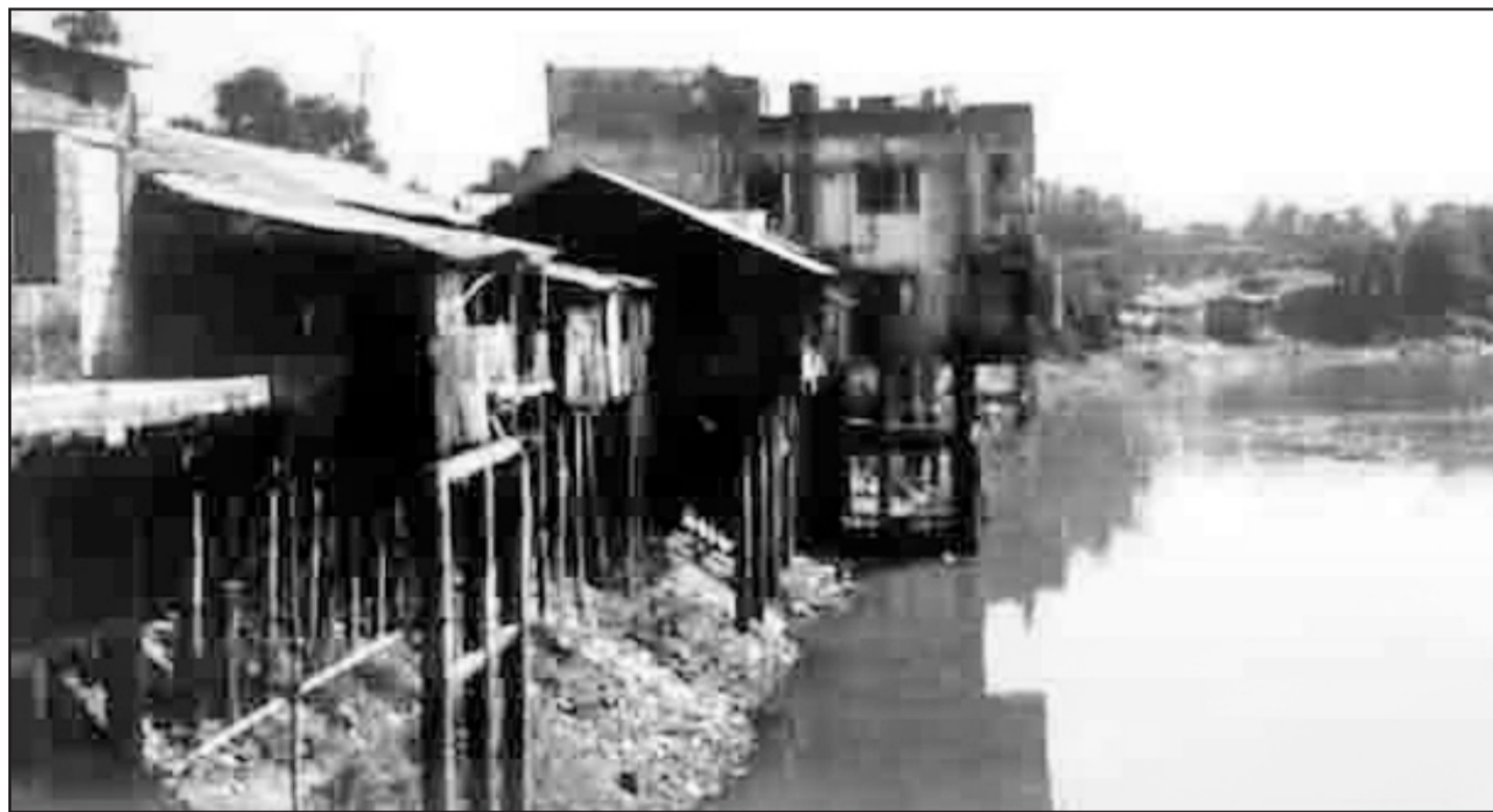
Unauthorised structures built by land grabbers on the bank of the Mogra in Netrakona town has squeezed the river.
