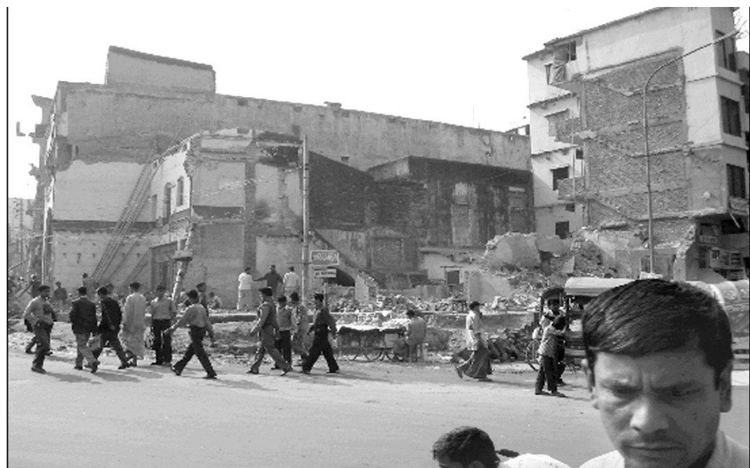
Road widening by demolition
