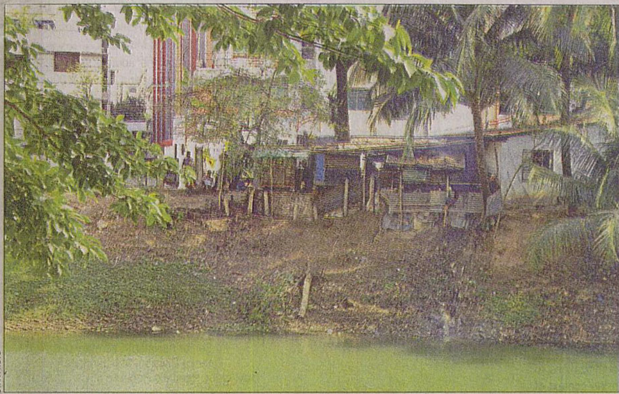
An illegal eating-house on the bank of the Dhanmondi Lake.
