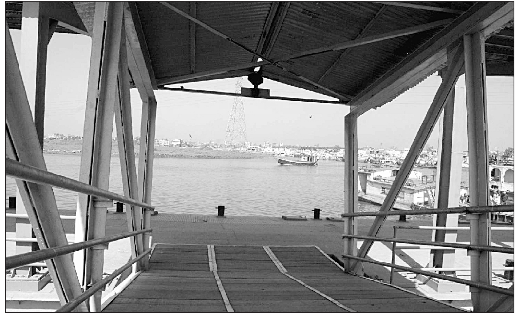
A landing station near Gabtoli to facilitate the water transport is almost complete (right).
