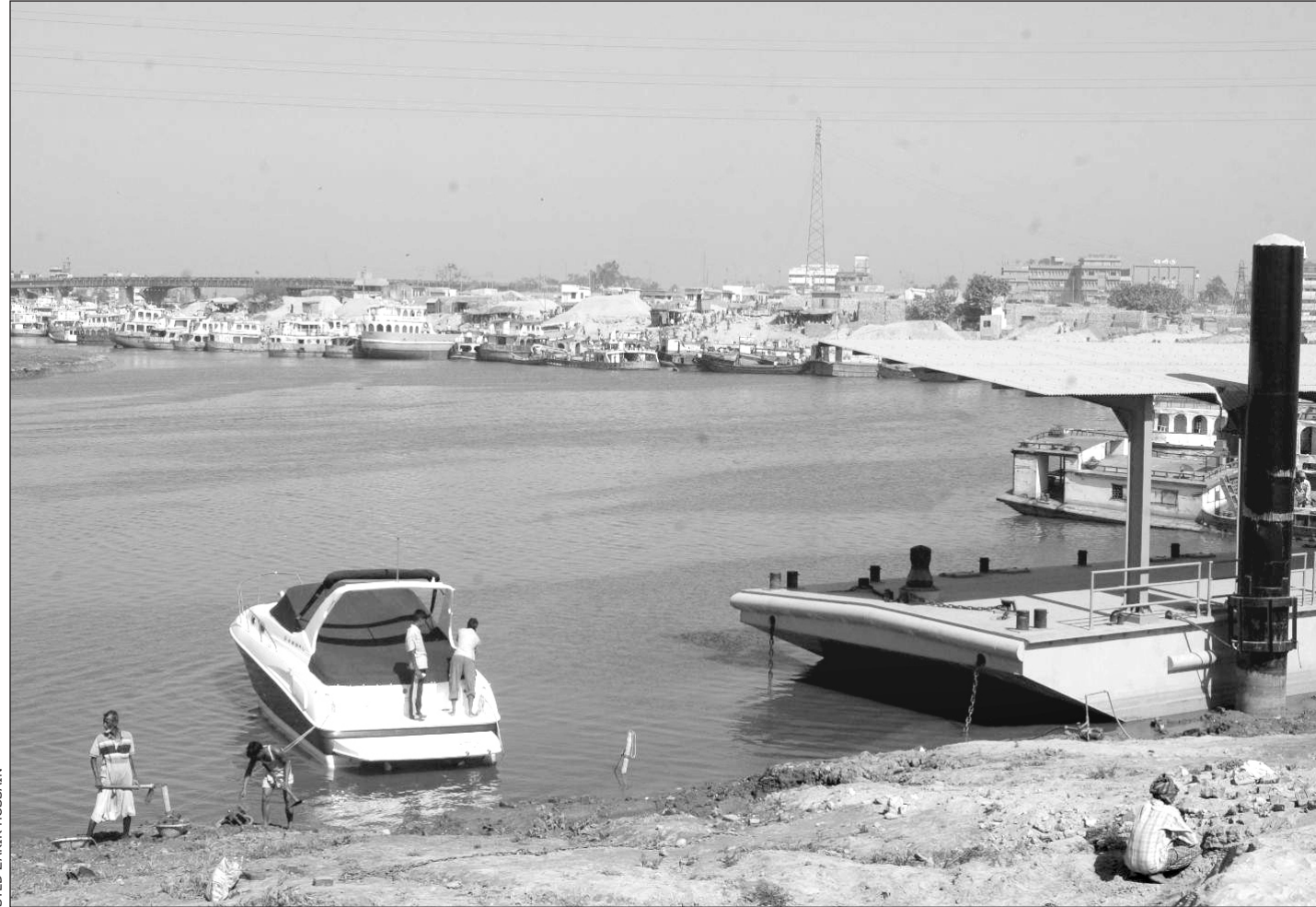
A section of the Circular Water Way project.
